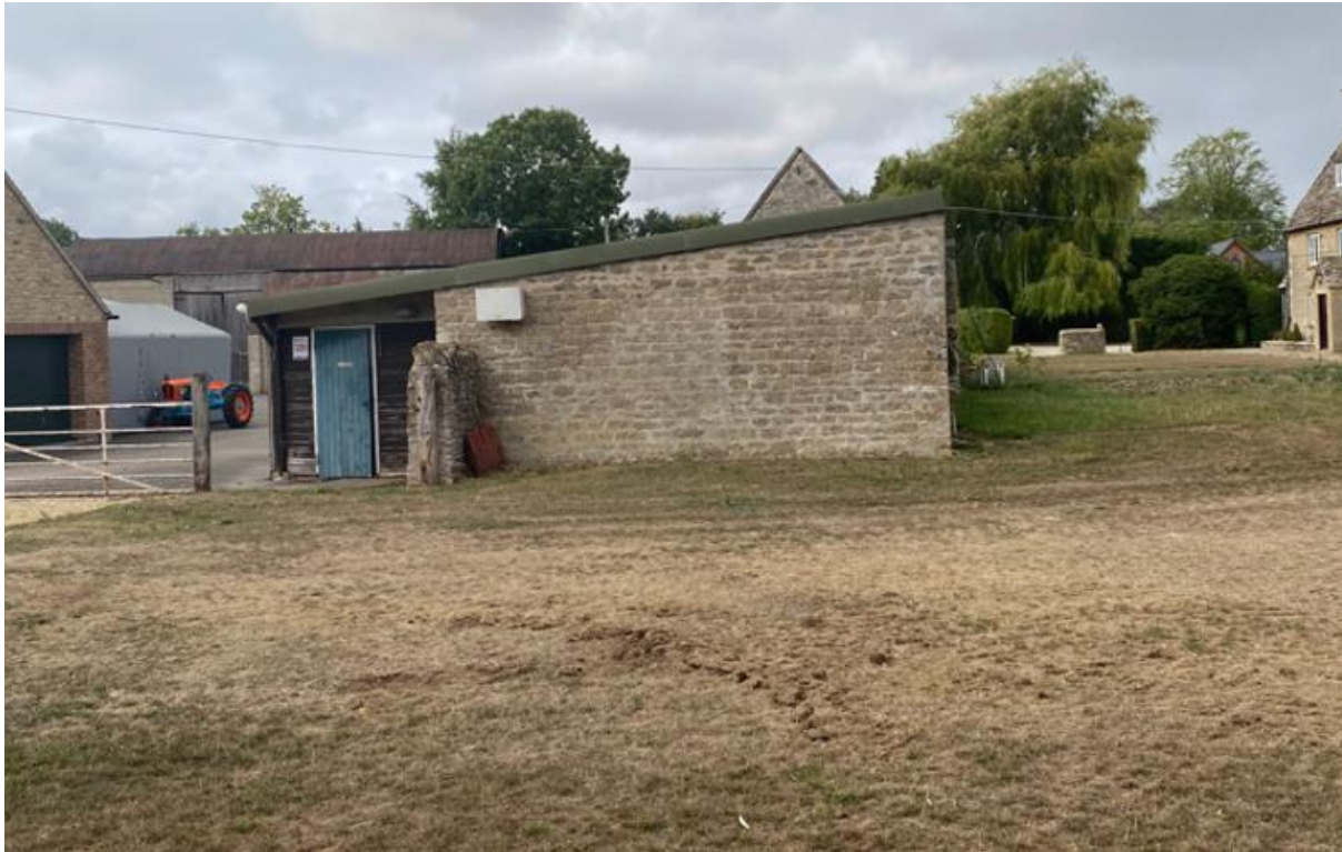
Side View of part of flat roof existing outbuilding (garages) to be demolished
