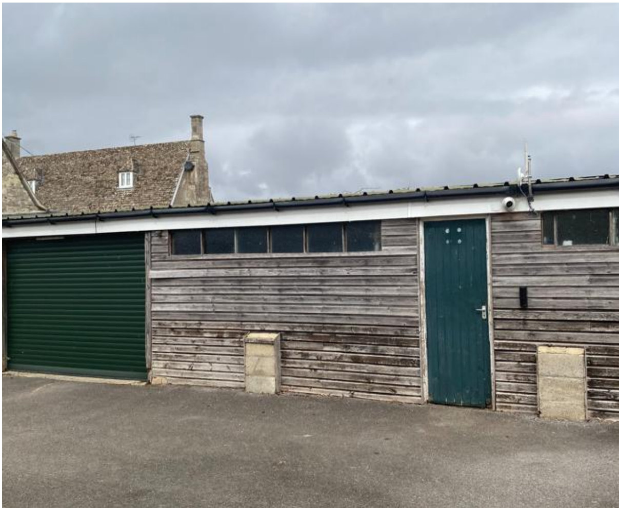
Front view of part of flat roof existing outbuilding (garages) to be demolished
