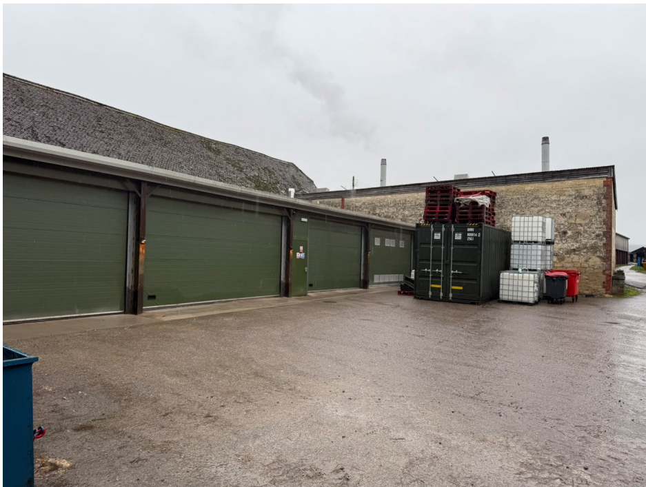
Photograph 4 – The lower courtyard with the modern extension to the listed building and the rear of the bio-mass building.
