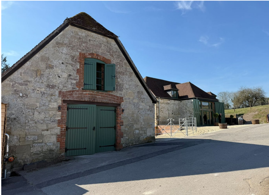
Photograph 1 – The converted barns as approved under applications PL/2021/10629 and PL/2021/10196.
