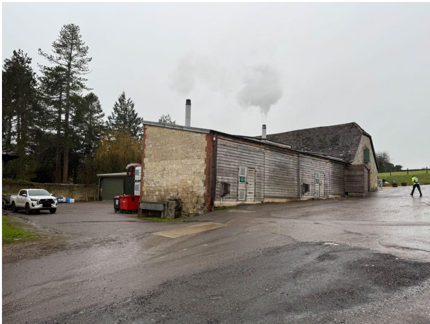
Photograph 2 – the bio-mass building and entrance into the lower courtyard.
