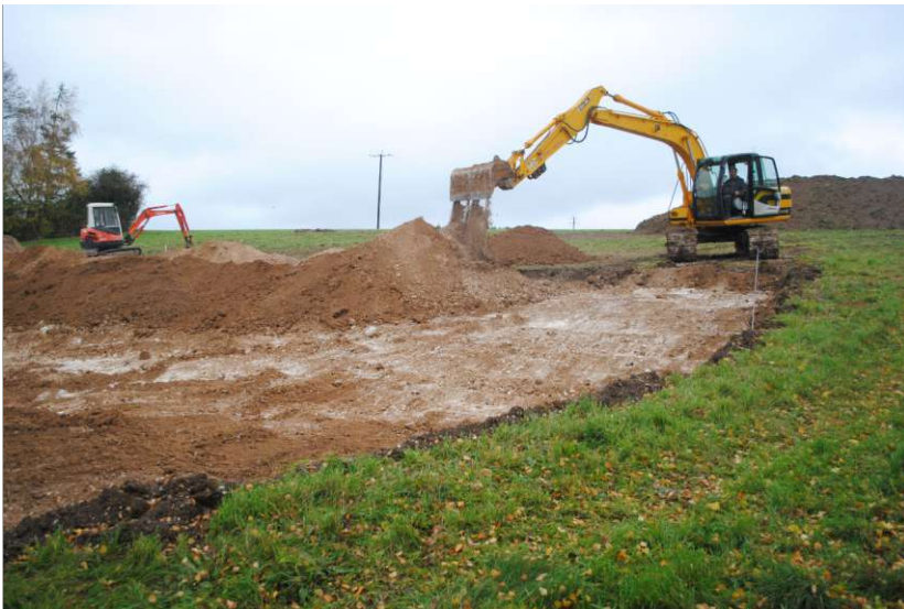
Plate 2: Working view during machine stripping of site. View to north
