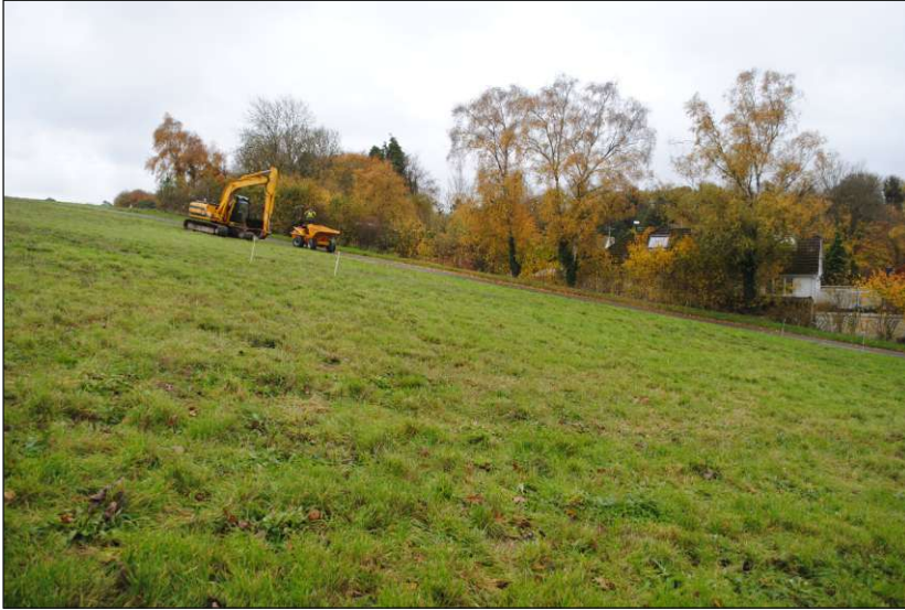
Plate 1: General view of site looking northeast
