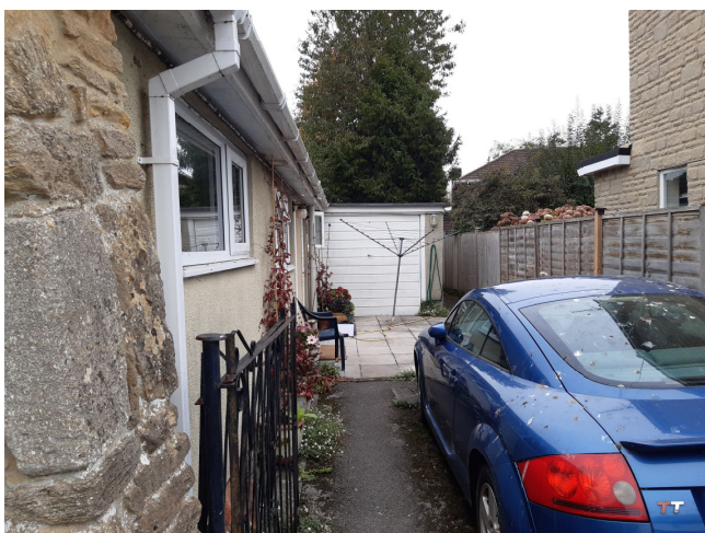
Site Photo 02. Existing South-West elevation of garage and South-East elev of house viewed from driveway.
