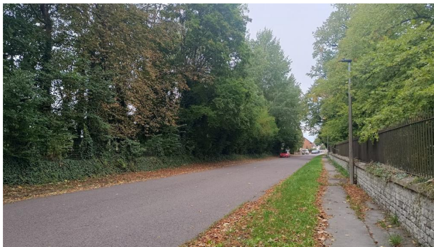
Figure 9: Photograph showing pavement opposite site entrance with streetlights along Park Street
