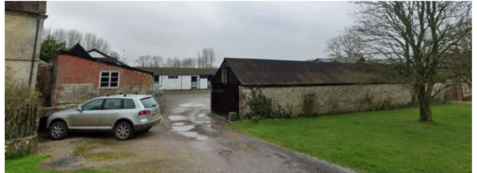
Typical courtyard of barns in a local village (Tytherington)
