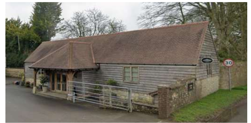
Timber clad converted barn – Tytherington
