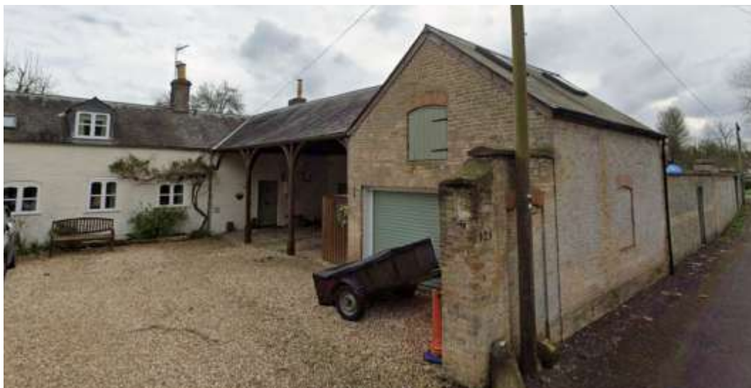
Brick & slate barn-like structures – Heytesbury
