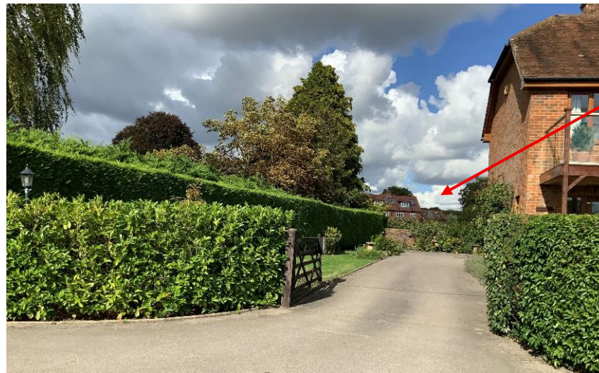
Image 3- western end of application site (above 1 st floor) would be visible. with rear of no. 1 Old Forge Close visible in the background
