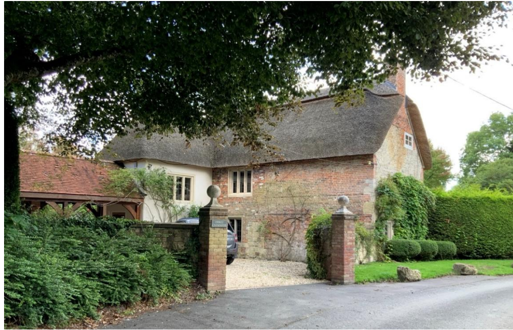
Three Chimneys entrance & driveway from Mantles Lane
