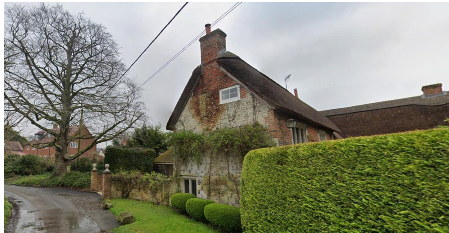
Looking north towards Three Chimneys with the back drop of Old Forge Close dwellings
