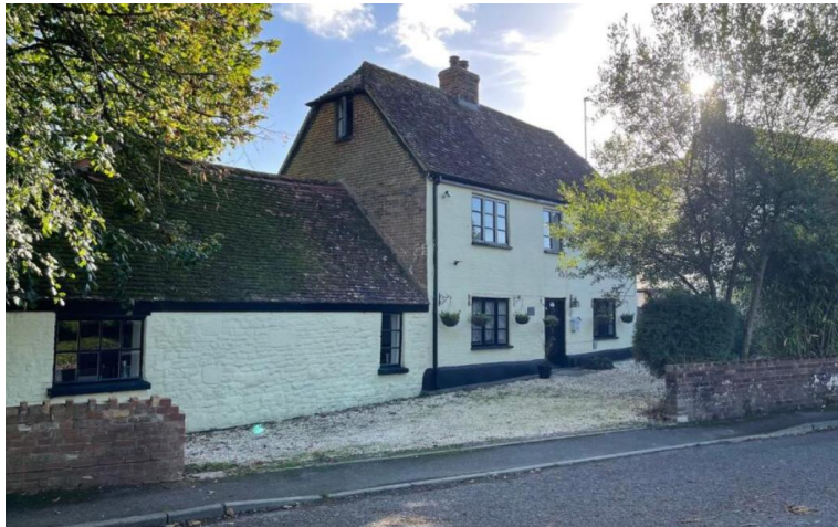
Tinkers' front elevation onto Park Street,
