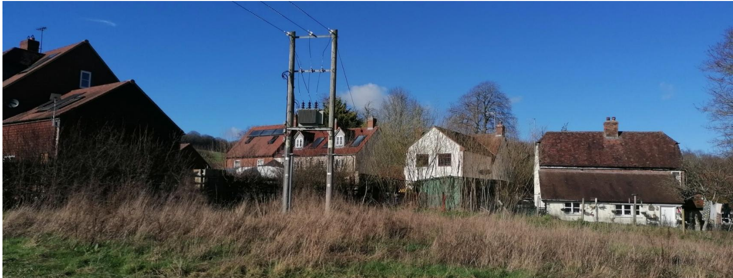
Photo of the rear of tinkers from the blue lined paddock to the south.
