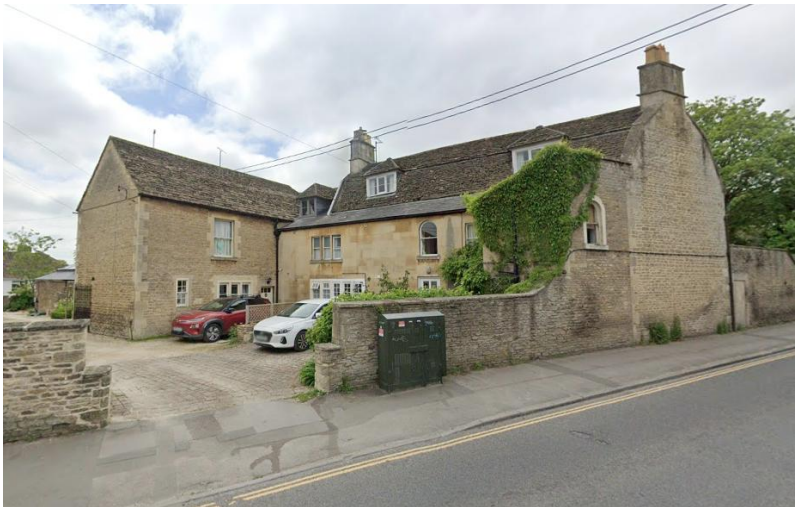
Front (North) Elevation (Google Image May 2023)
