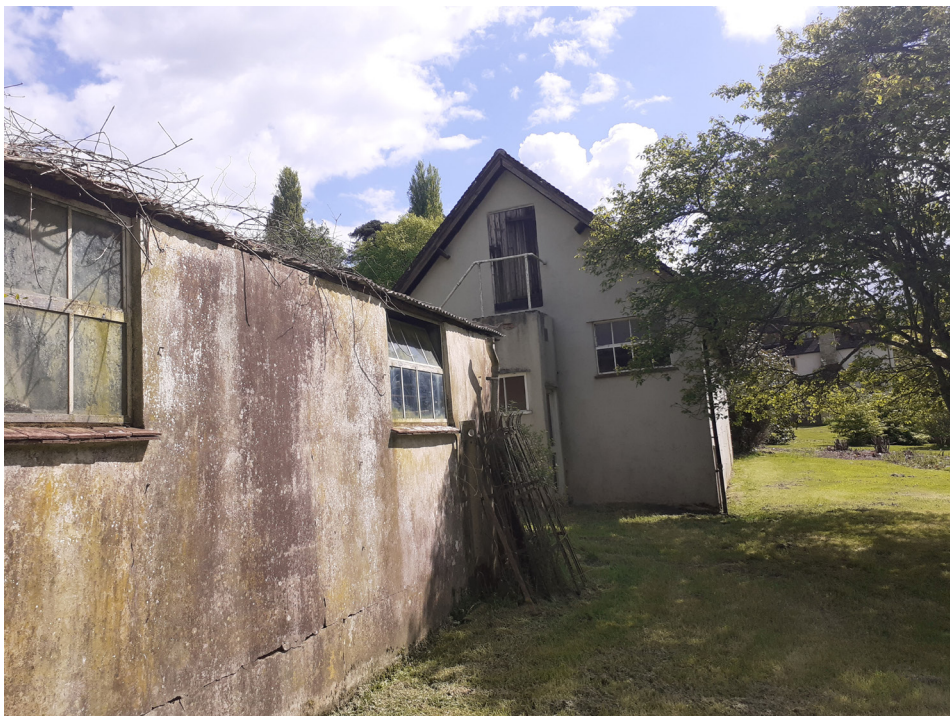
View of the existing ancillary accommodation with storage out building
