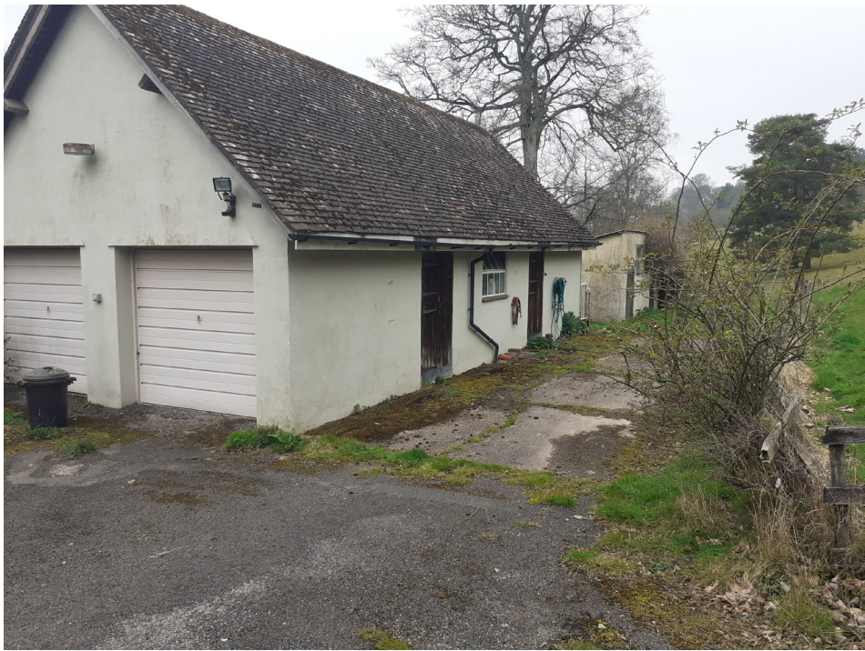
View of garage and ancillary accommodation
