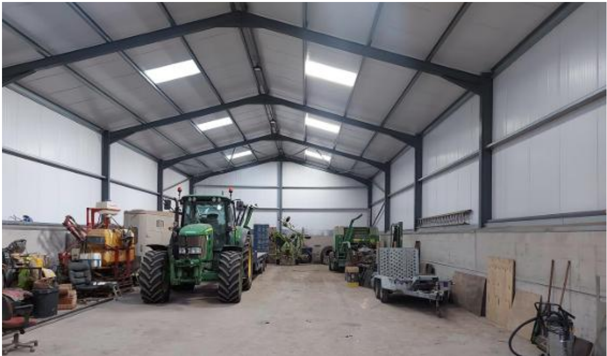
Figure 4: Building interior (source: Applicant's Planning Statement).
