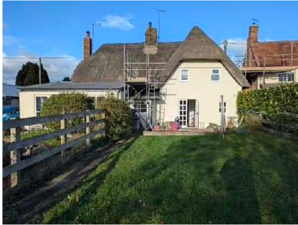
2. The rear elevations showing the extension to No.15 and the gabled elevation of No.14
