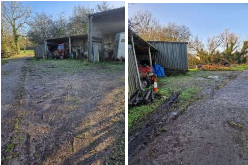
Photographs 1-3: Western area – Building & hardcore surface
