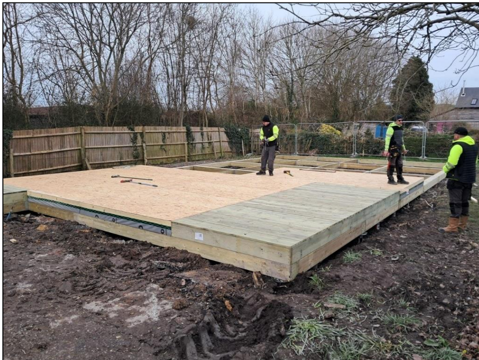
Picture 4: The shop being built off a ground beam
