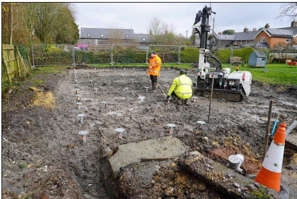
Picture 3: Ground screws being installed
