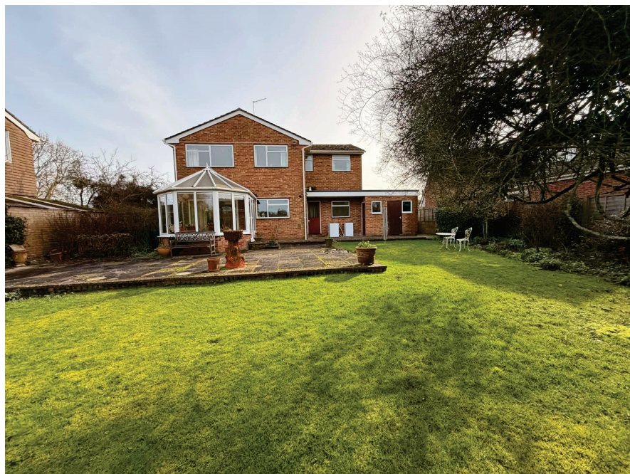
Photo 2 – Rear of property looking at existing building.
