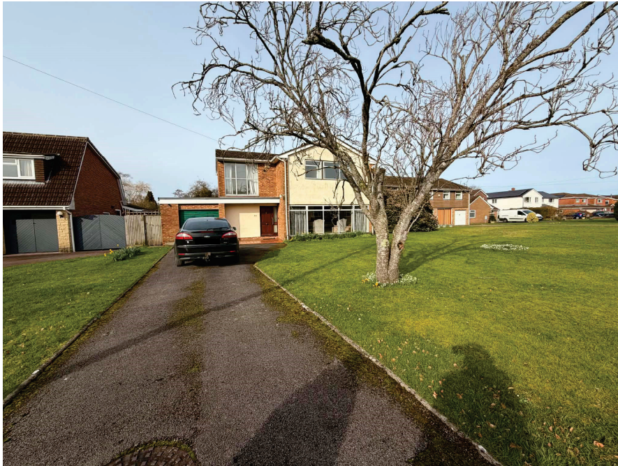
Photo 1 – Front of property.
