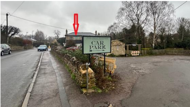
Below: Car park and rear elevation – existing gable board shown by red arrow.
