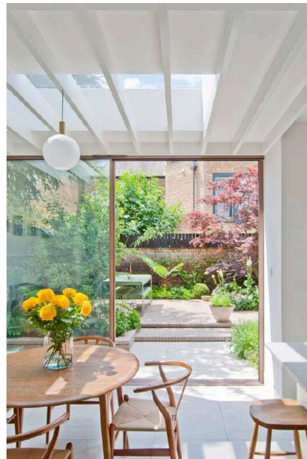
Painted joists usual when relying of more standard timber.
