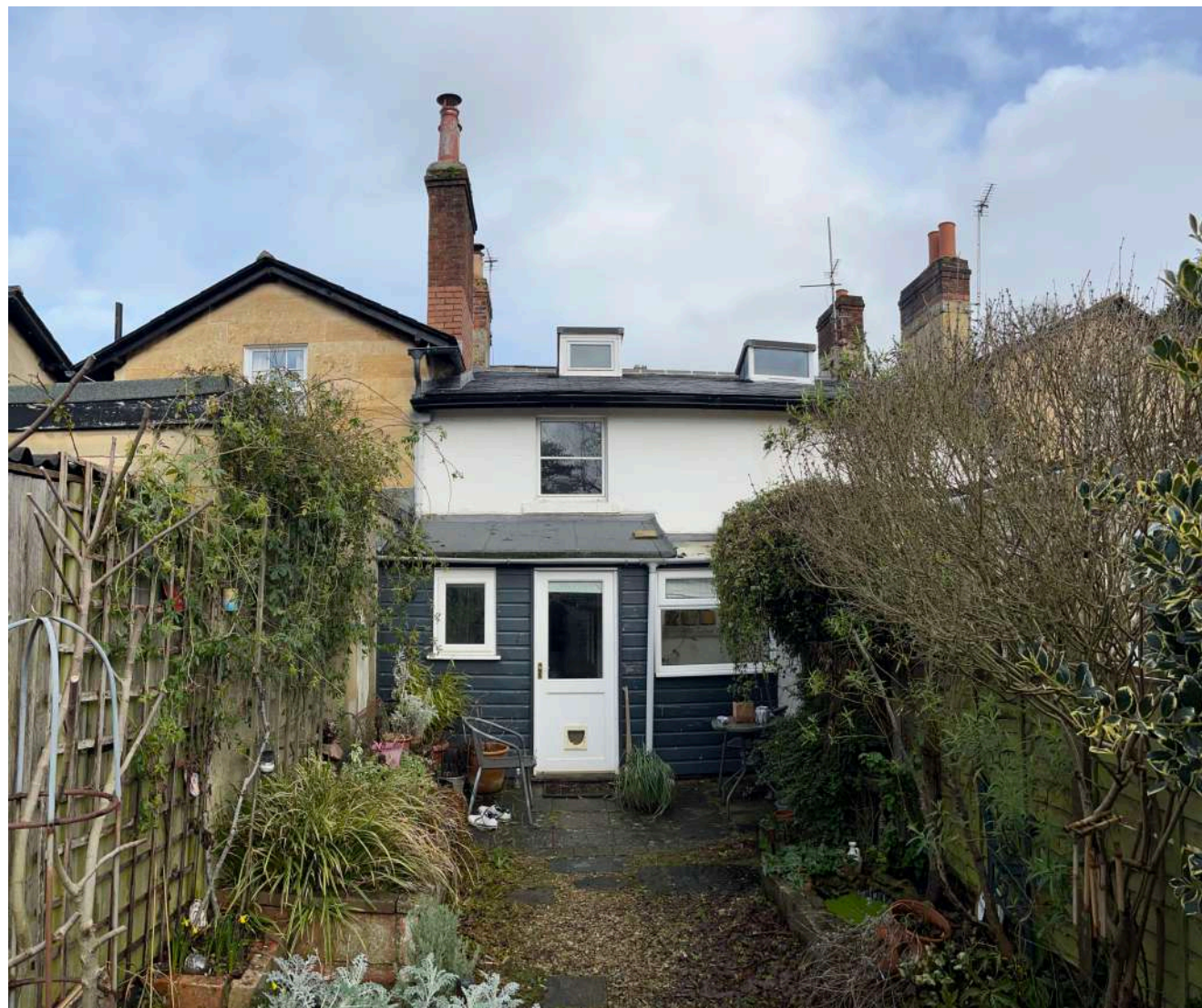
Existing rear view with lean-to extension to be removed.
