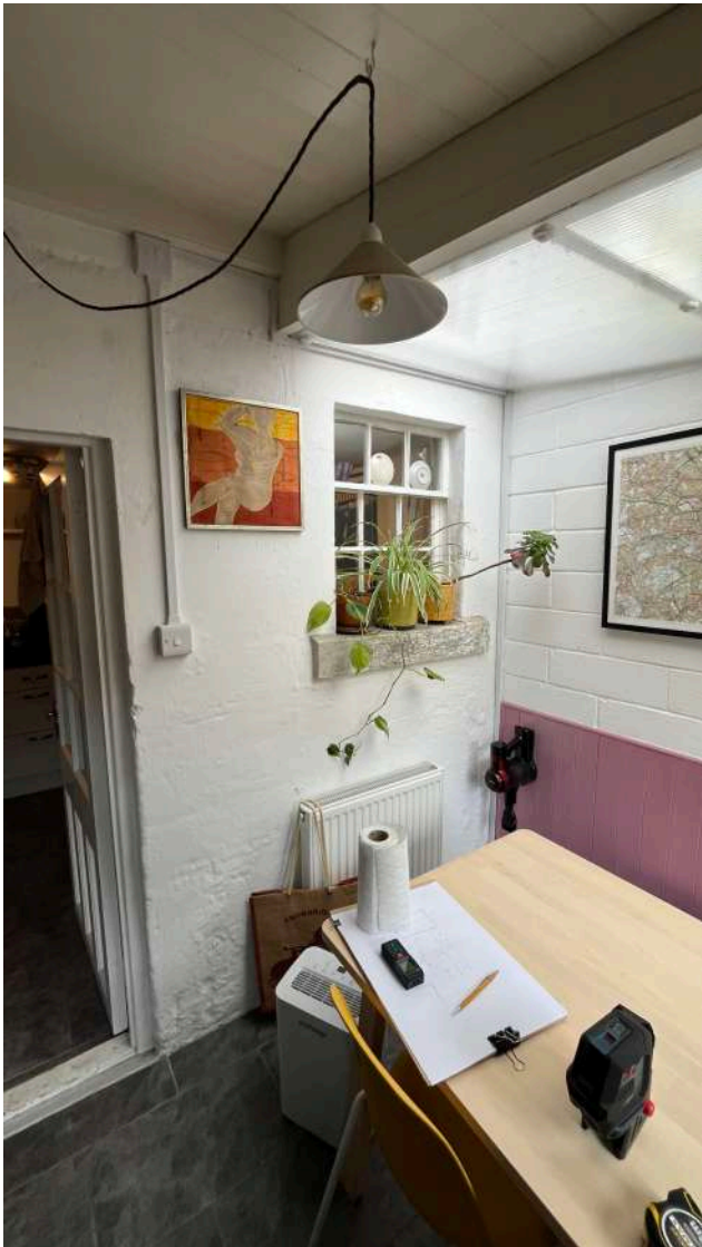
Historic window to be retained
