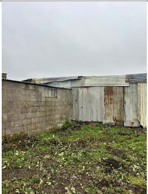
Barn 4 Rear (Southern) Elevation
