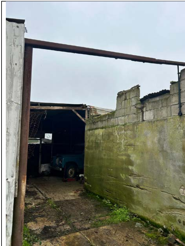
Barn 4 Front (Northern) Elevation
