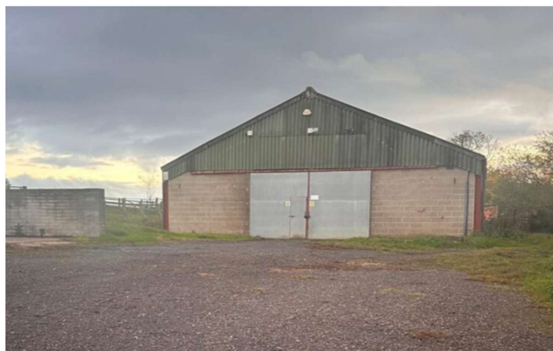
Figure 1: Principal elevation of barn at site.
