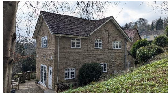
Photograph 4: The northeast gable and northwest elevation of B1.
