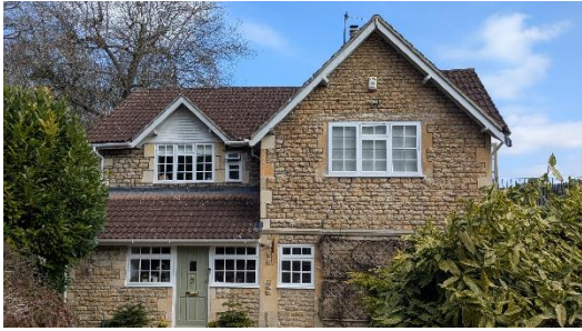
Photograph 1: The southwest elevations of B1.
