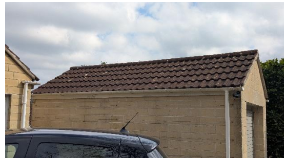
Photograph 20: Northwest roof pitch of B3.
