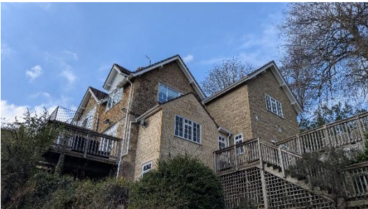
Photograph 3: The northeast elevations of B1.
