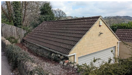
Photograph 15: Northwest roof pitch of B2.
