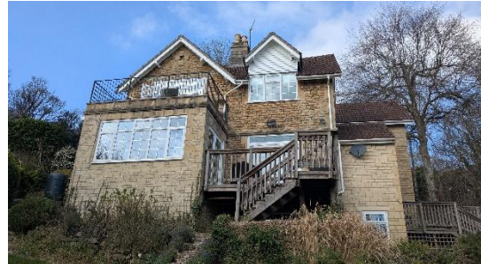
Photograph 2: The southeast elevations of B1.
