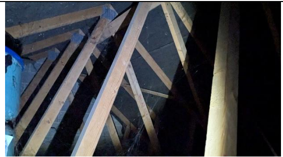
Photograph 18: Small loft space at the northern end of B2.
