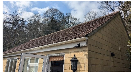
Photograph 16: Southeast roof pitch and northeast gable of B2.
