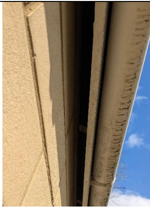
Photograph 17: The gutterboard of B2 sitting far from the external wall.
