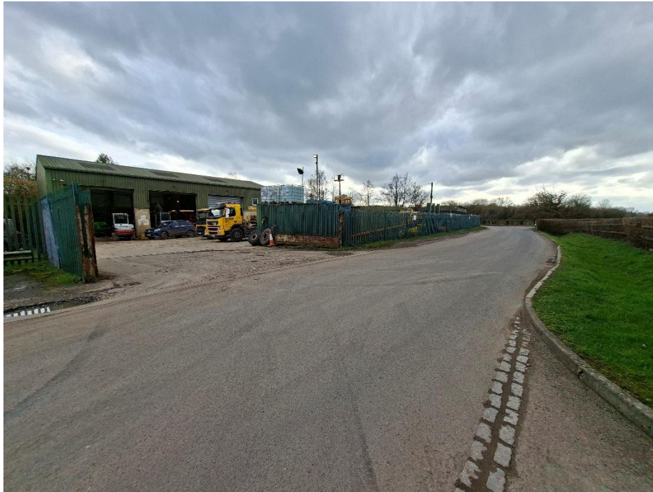
Figure 4: Existing Coppard Plant Hire site
