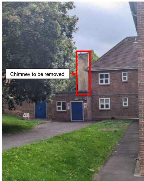
Photo 1 – Showing the chimney to be removed.
