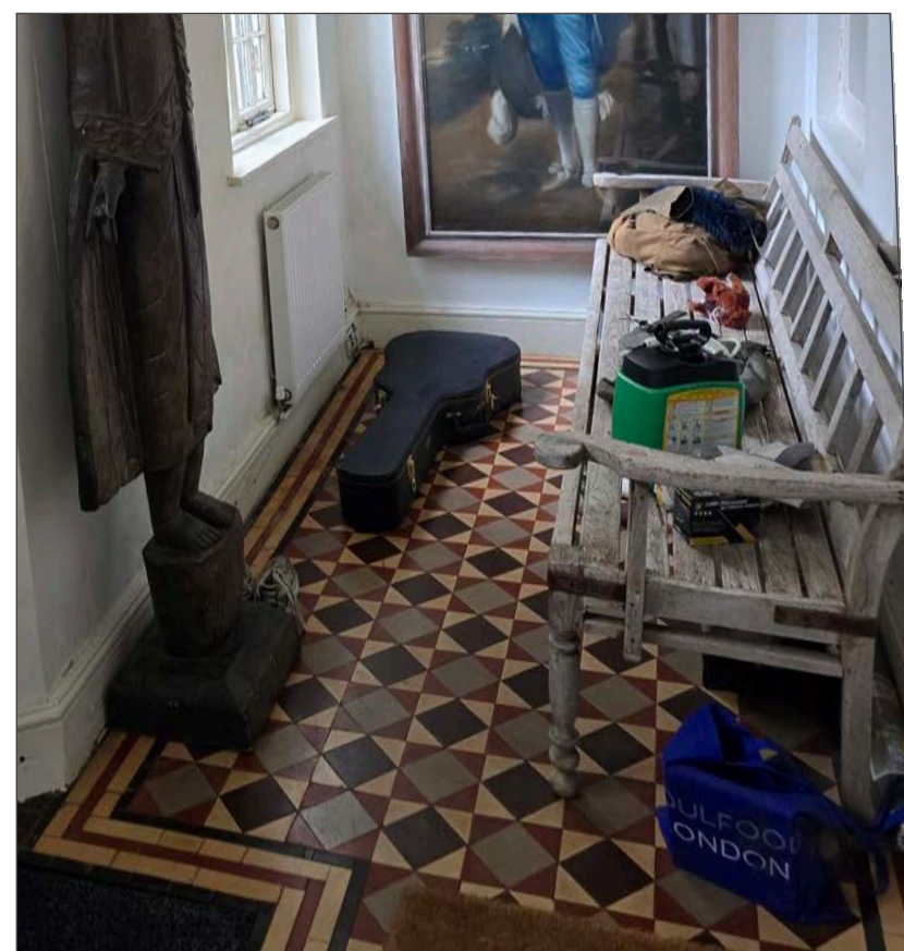
Figure 31: modern tiles floor to be replaced with stone flags
