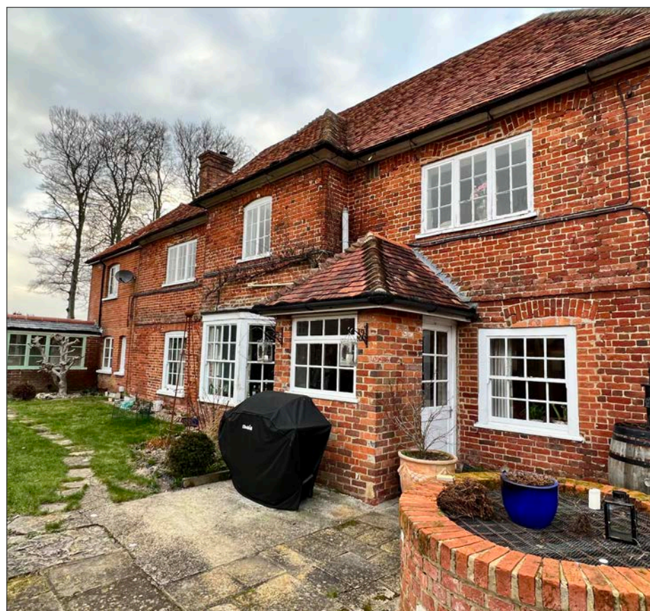
Figure 10: fenestration altered at rear ground floor, brick arch heads with later inserted sashes. Modern small boots room addition.
