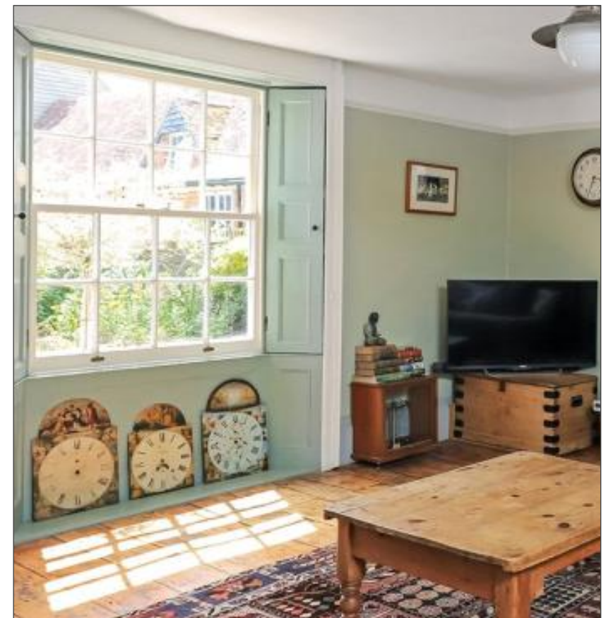
Figure 16: early to mid 19th century joinery and window shutters
