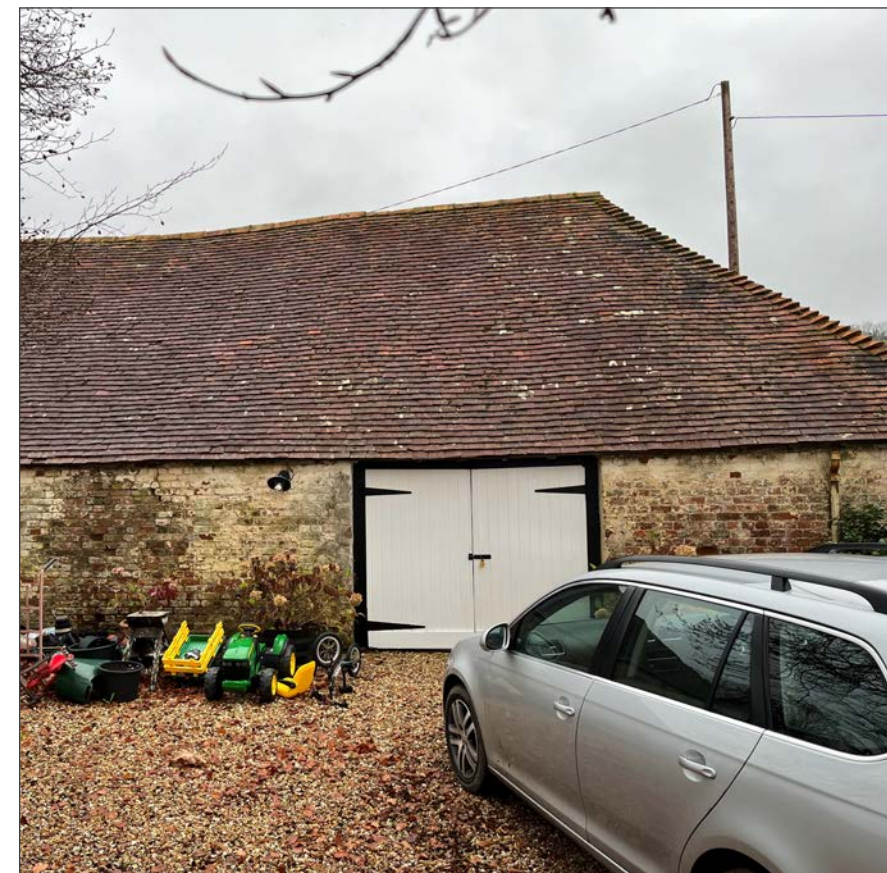
Figure 8: brick building with hip roof is the grade 2 cart-shed
