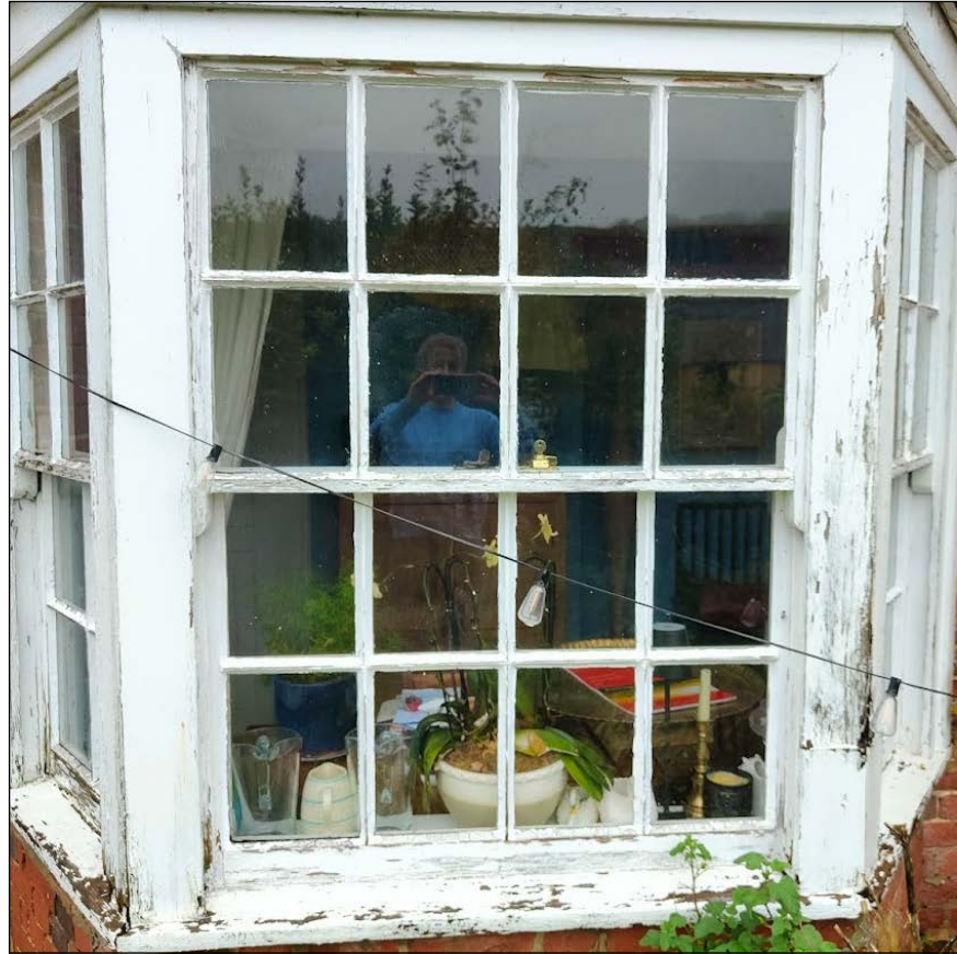
Figure 23: W31 bay which is to be replaced with the exact joinery detail, glazing bar mouldings and salvaging the heritage glass.
