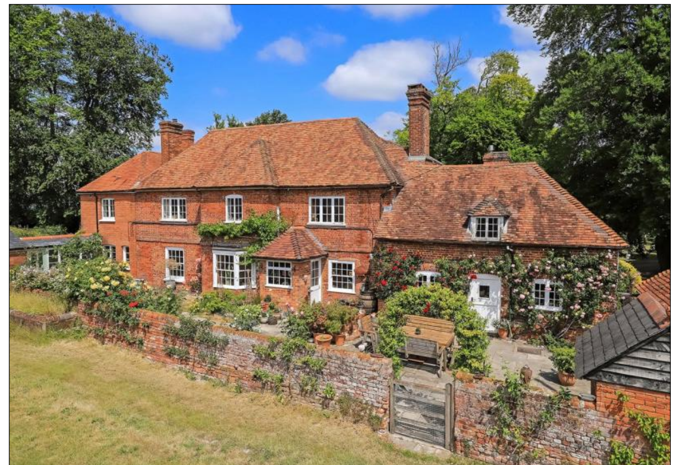
Figure 2: Rear south elevations which remain in exposed brickwork
