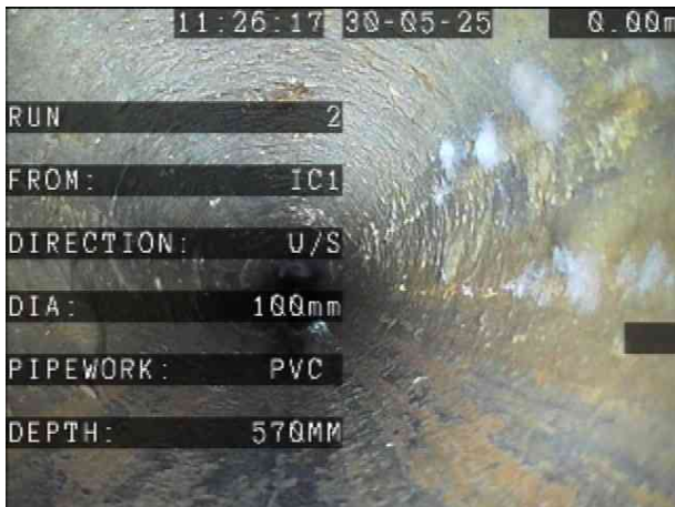
InternalX_eb514271-c333-4e0a-9e8a-d3de86de49fa_20250604_131243_093.jpg, 00:00:00, 0.00 m Start node, inspection chamber, reference: IC1
