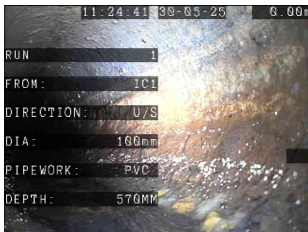
W.C.X_86f5473a-15ae-4514-9074-cabb1a888ccc_20250604_130658_383.jpg, 00:00:00, 0.00 m Start node, manhole, reference: IC1
