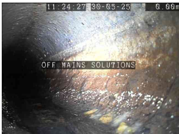
W.C.X_eaa3eb21-041d-444a-95fb-eb485c41235c_20250604_130650_605.jpg, 00:00:00, 0.00 m Start node, manhole, reference: IC1
