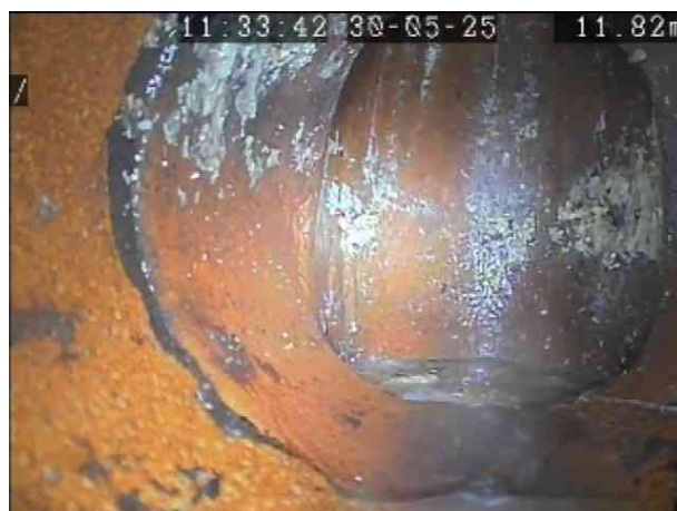
IC1X_4f8c3061-1447-415c-b93c-235797a514f6_20250604_13 2827_211.jpg, 00:00:44, 11.82 m Finish node, catchpit, reference: Septic Tk
