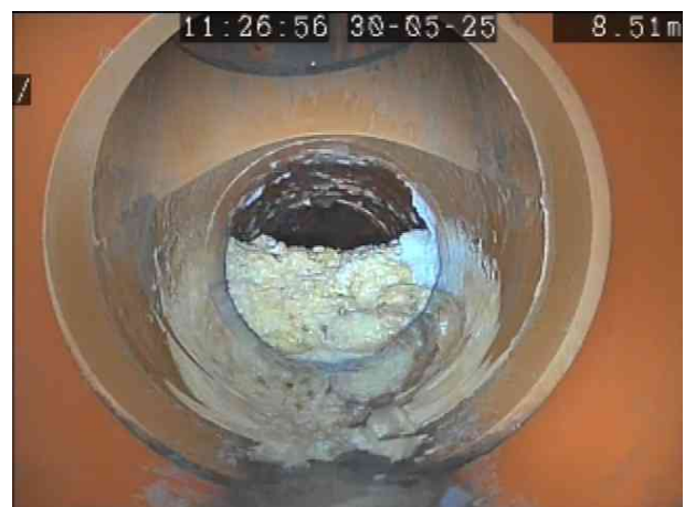
InternalX_546a6515-bc16-4f24-bafc-8bc8a2373bb8_20250604_131424_633.jpg, 00:00:39, 8.50 m Junction at 12 o'clock, 100mm dia
