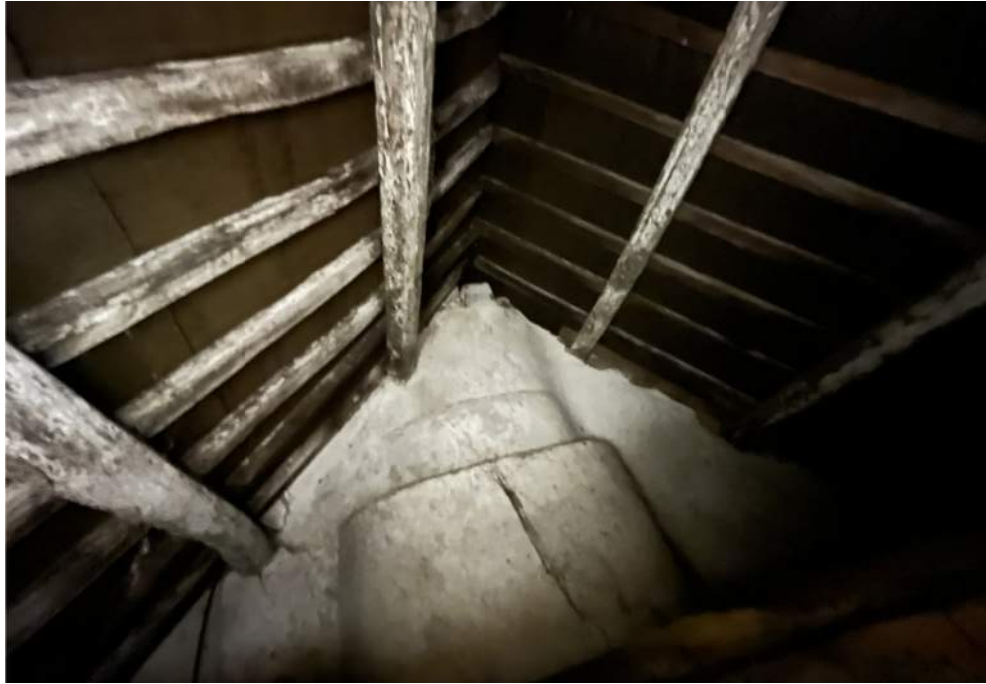
11: View into loft over tap room - note chimney flue
