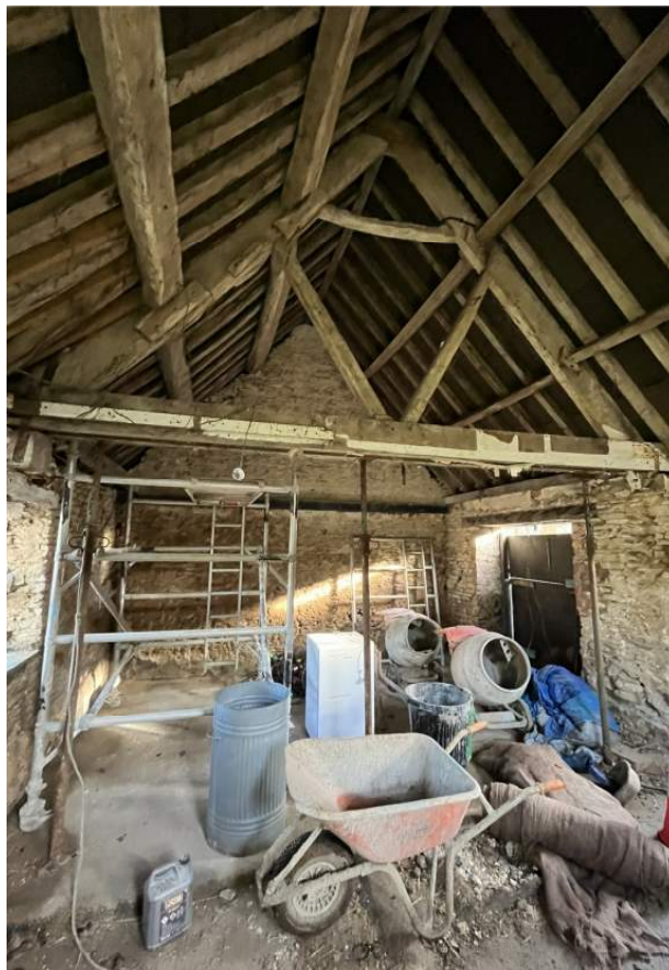
4: Internal view within store 1 looking northeast
