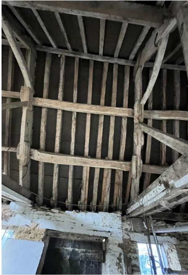
5: Section of roof with older purlins and common rafters
