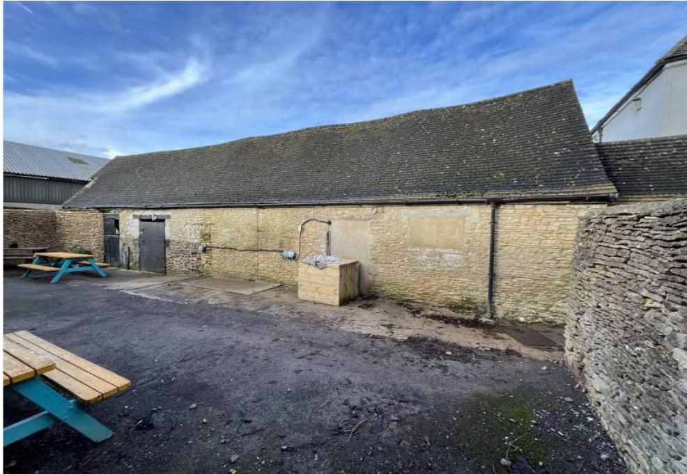
1: View of main barn building from south east
