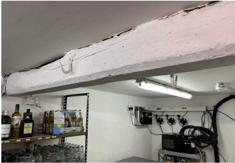
9: Tie beam to timber truss in tap room
