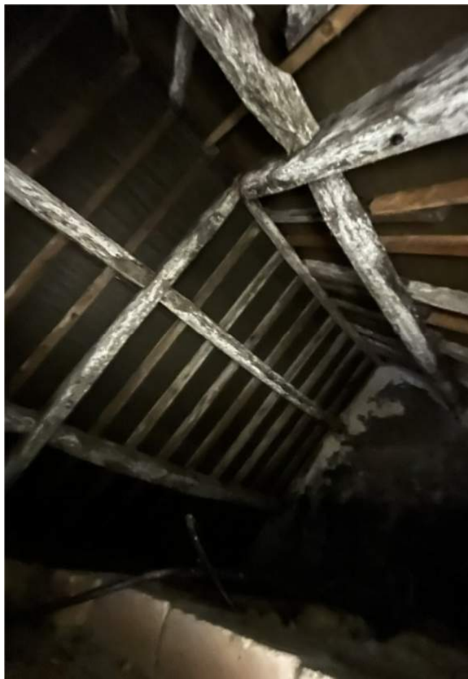
10: View into loft over tap room - white on timbers to be checked but most likely to be paint
