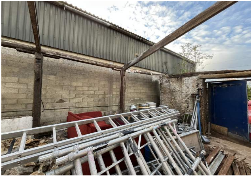
15: Views of west side to store 2 showing timber framing to removed pitch roof
