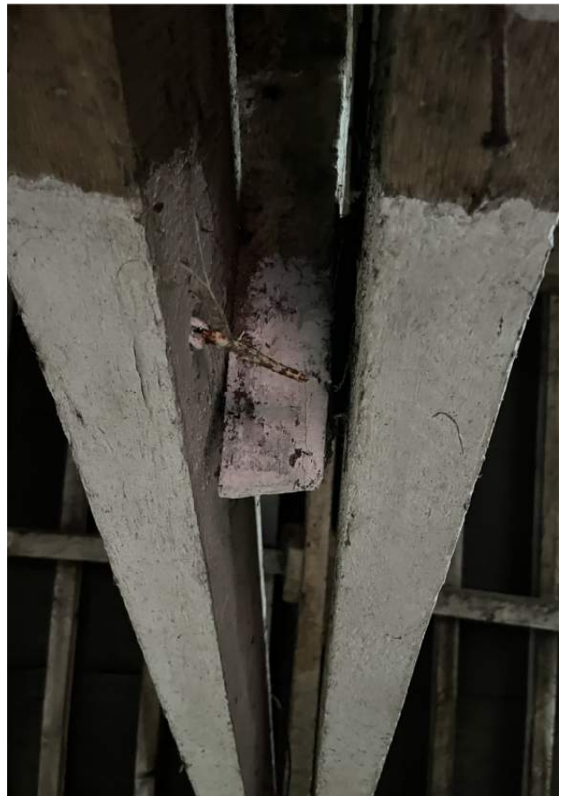
8: Alterations to the timber trusses - original tie beam cut and replaced with a pair of timbers. Diagonal struts are not properly attached to tie beam
