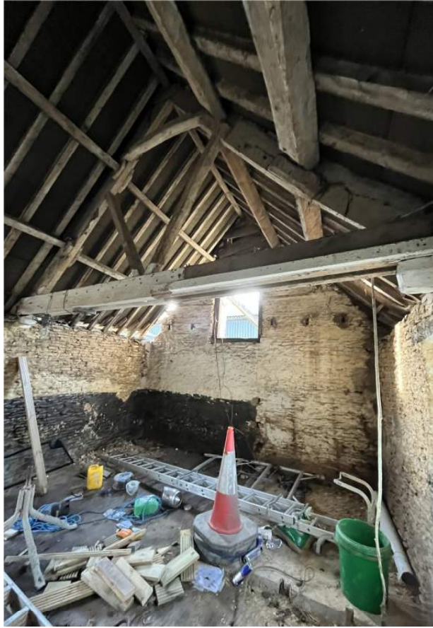
3: Internal view within store 1 looking southwest (dividing gable wall with store 2)
