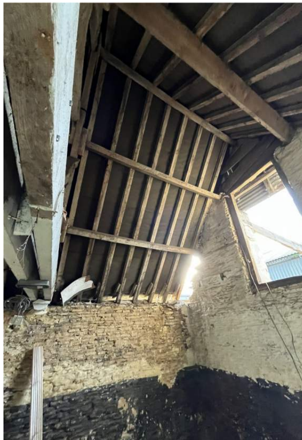
6: Section of roof with more recent purlins and common rafters
