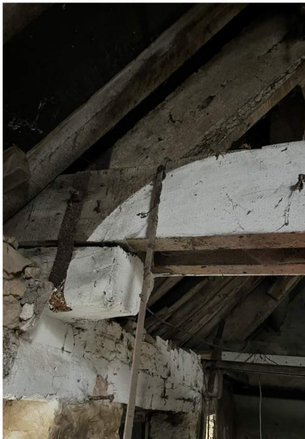
8: Alterations to the timber trusses - original tie beam cut and replaced with a pair of timbers. Diagonal struts are not properly attached to tie beam
