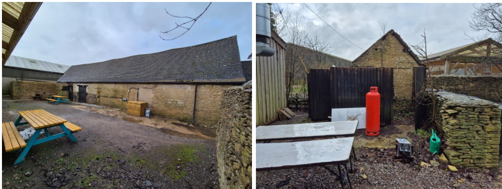
Further view to rear of barn where outdoor bar has been removed and separate outbuilding (to be used as spa plant building) alongside timber boarded northern end to the function building.
