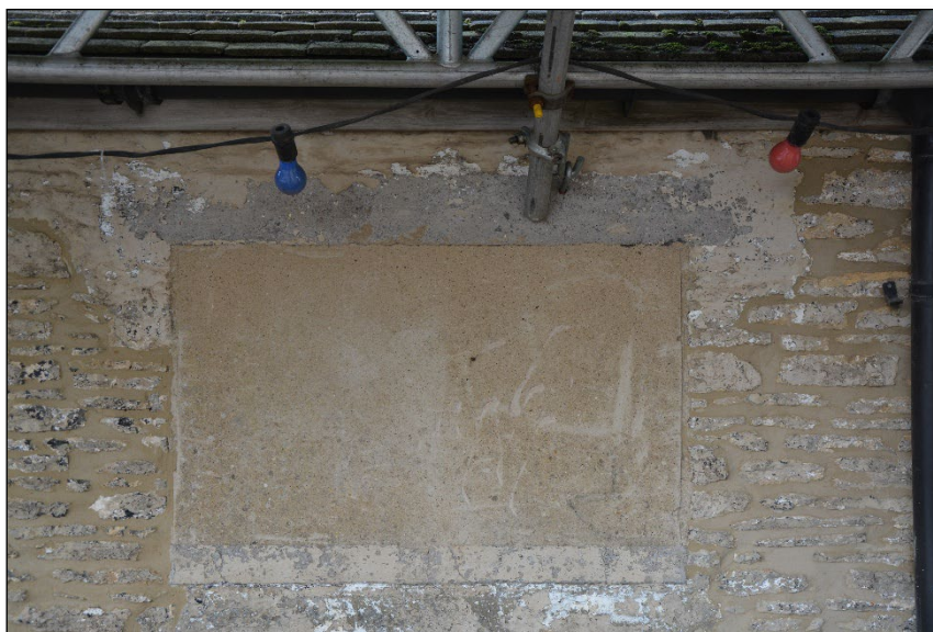
Image 14: Blocked opening, south elevation
