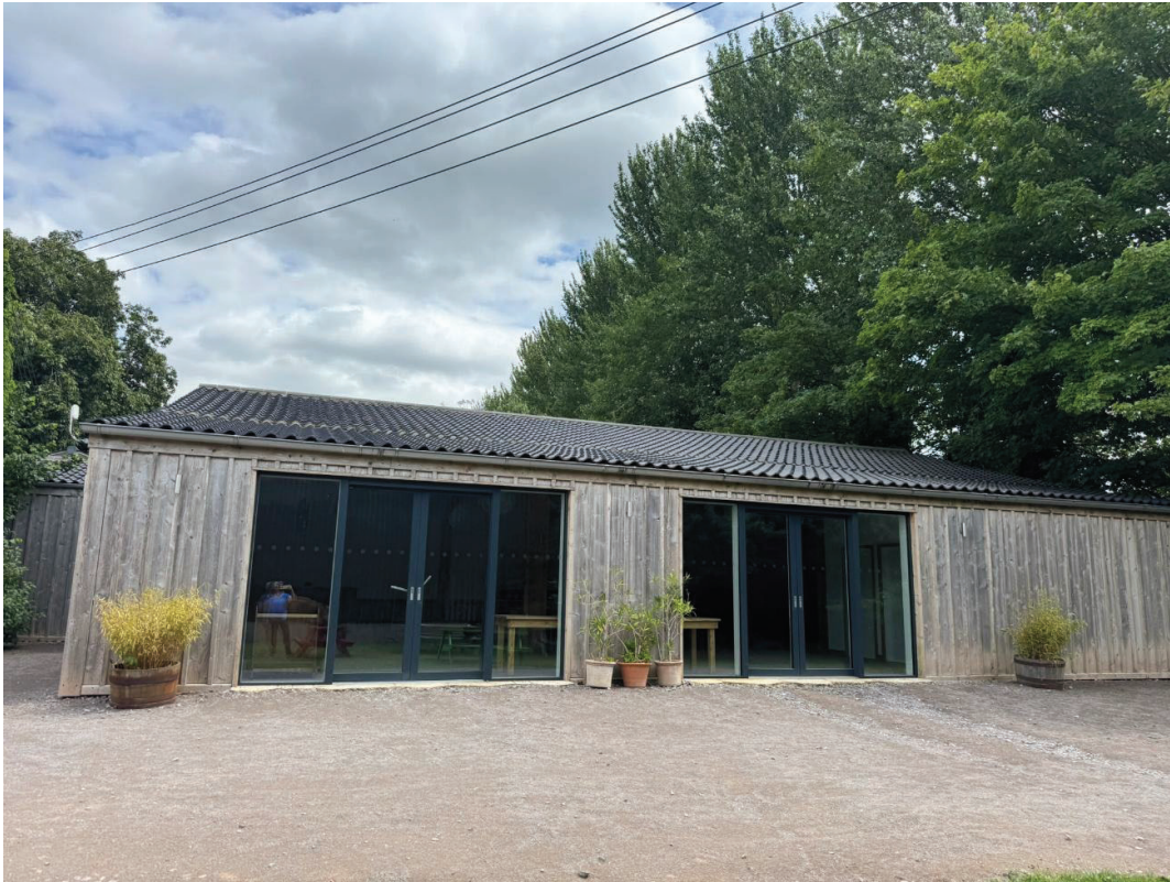
Plate A3 Modern Function Building showing area where the extension is proposed
