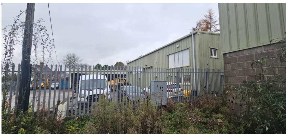
Above: Workshop building (right) and adjacent buildings at C & G Surfacing (left)
