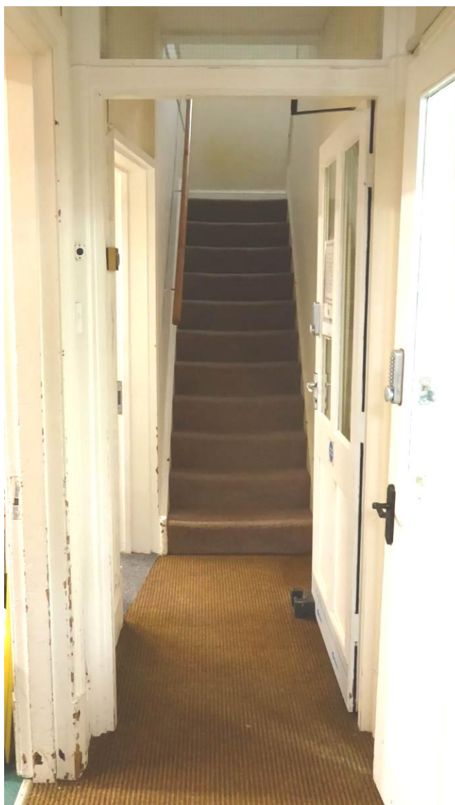
Fig 3.2.2: Existing ground floor travel route and stairs to first floor
