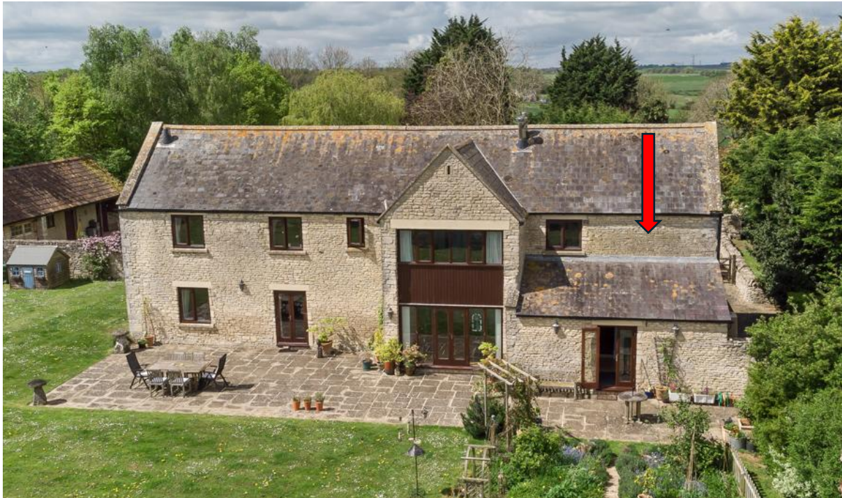
Fosse Barn rear (West) elevation – Location of proposed works highlighted
