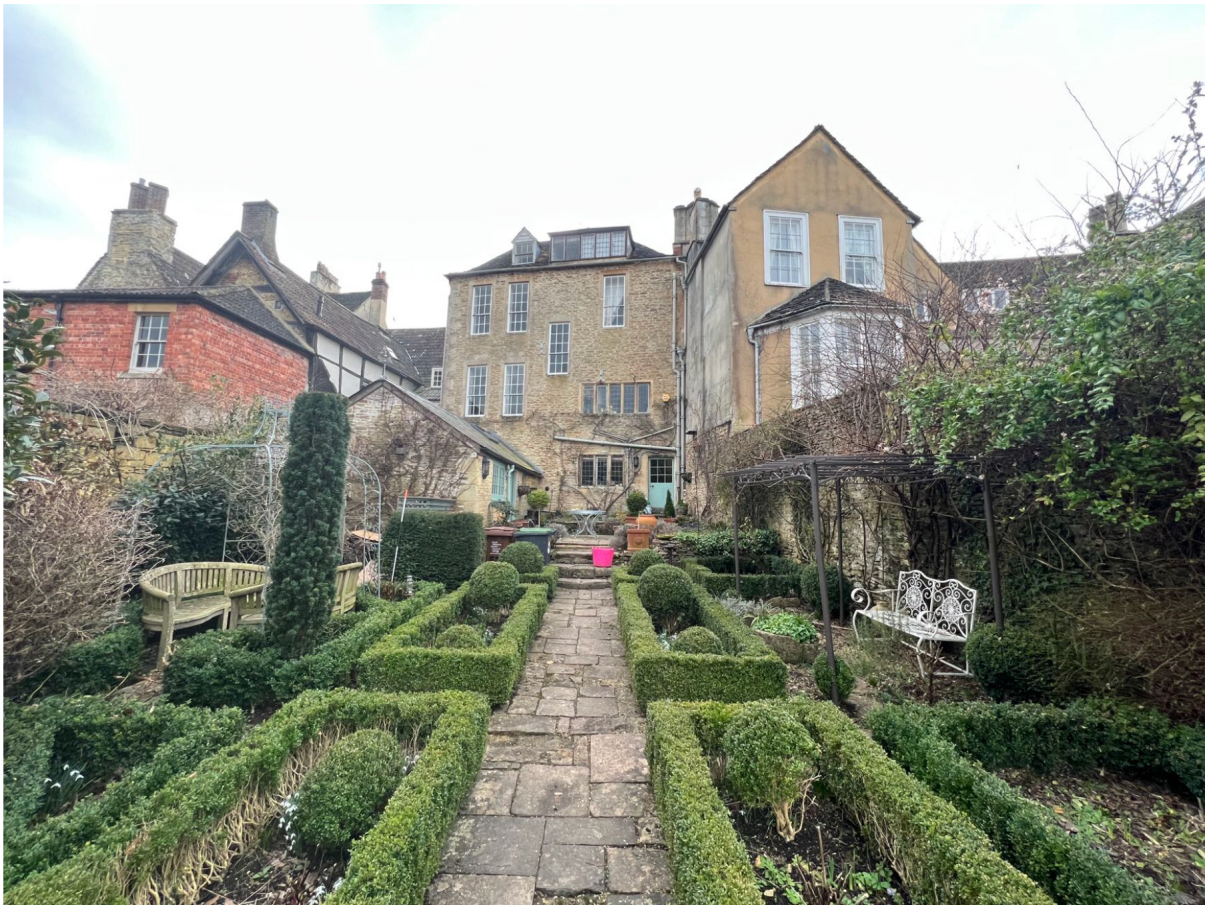
Rear elevation of Zealys House - 53 St Mary Street
