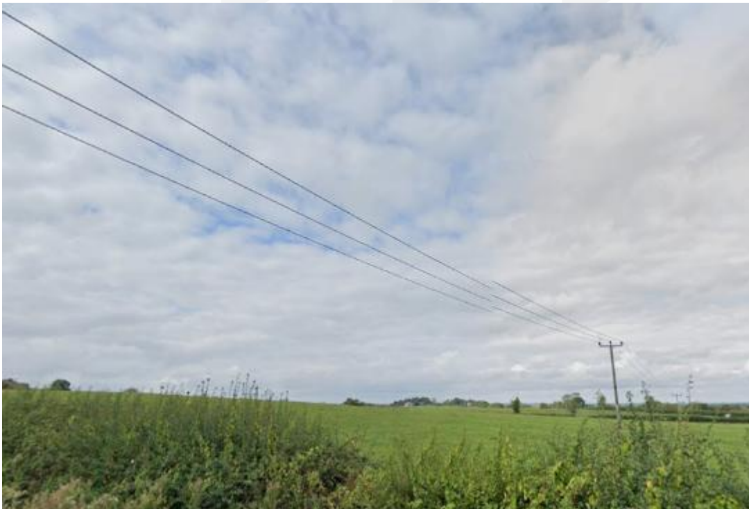
Image 1: Existing 33kV EHV Cables (source Google Earth)
