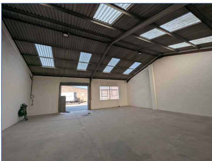
Figure 4. Internal view of Unit 21 (March 2026)
