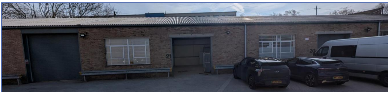
Figure 3. External view of Unit 21 (March 2026)
