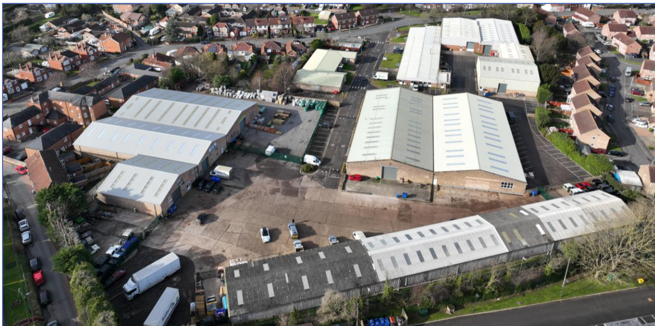
Figure 2. Drone Photograph of the application site – Unit 21 is located in the rank of buildings in the foreground. NB. this photograph predates the white lining of parking spaces on the site.
