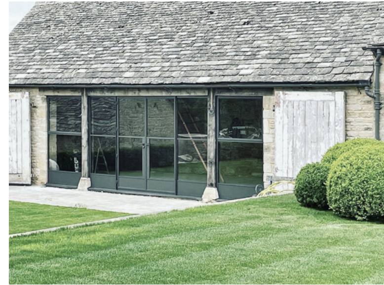
Example of crittal style glazing with timber posts and saddle stones
