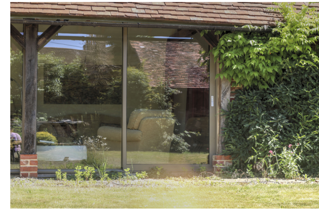
Example of glazing set behind structure
