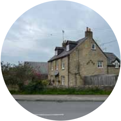
2.5 storey home defining key junction in Cricklade
