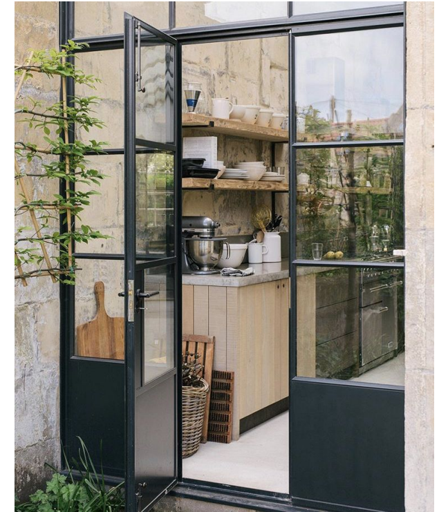
Example of crittal style glazing in lean-to
