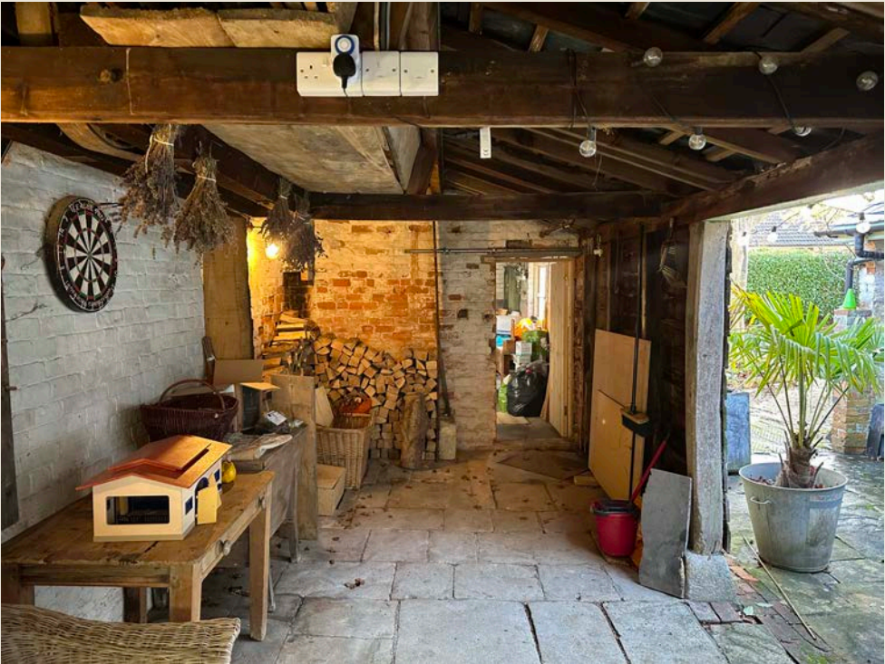
Figure 1- The existing store, leading through to the garage and courtyard
