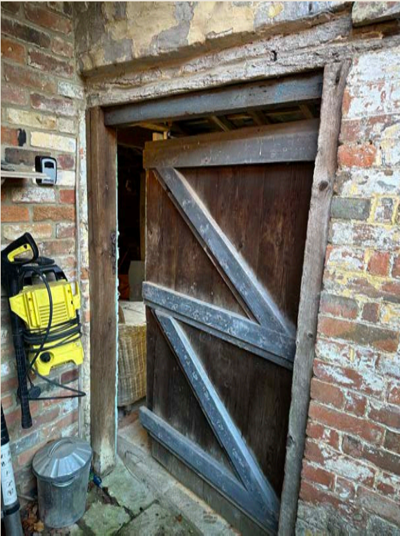
Figure 8- Existing ledged and braced door/gate between rear garden and store
