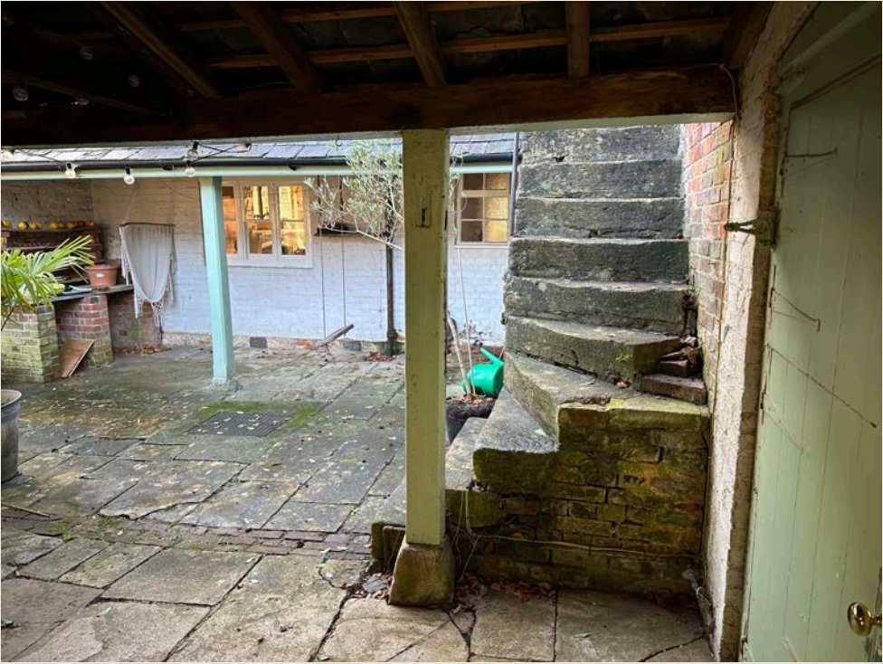
Figure 2- View onto courtyard from within existing store
