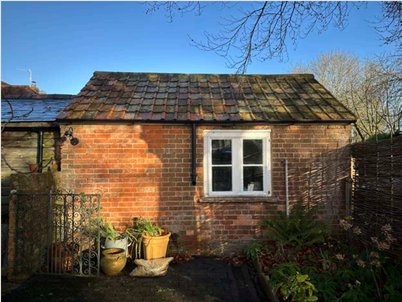
Figure 12 - South elevation of existing garage
