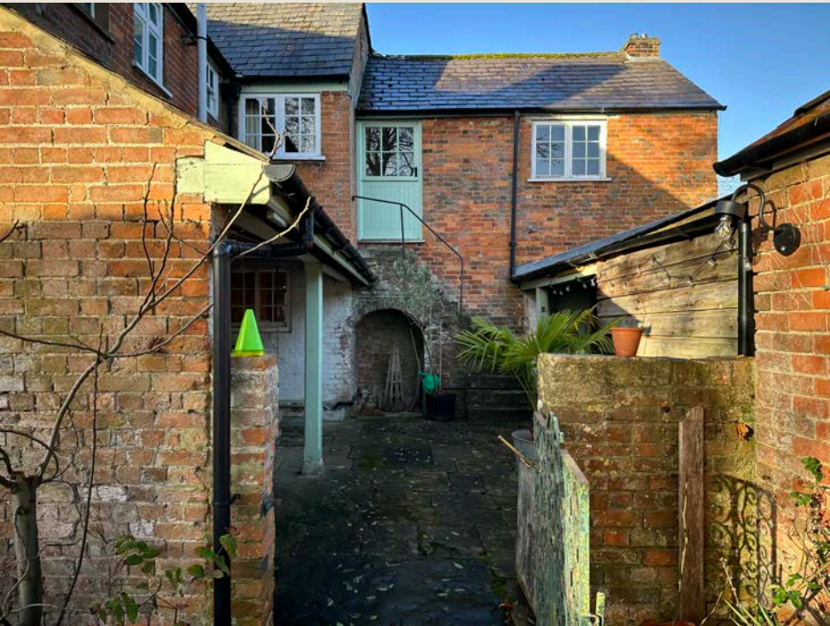
Manor House courtyard and associated outbuildings/garages, 2025
