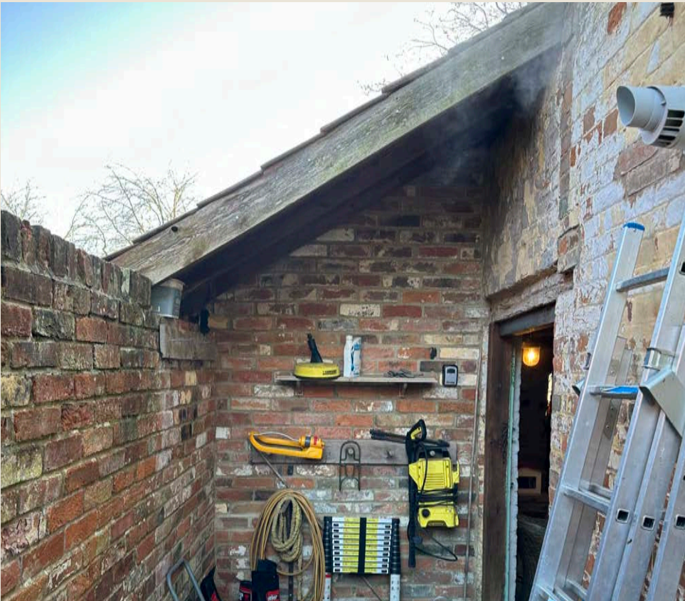
Figure 6- West elevation of the store, roof overhang forms neighbouring property's outdoor store. Door connects rear garden with the store.
