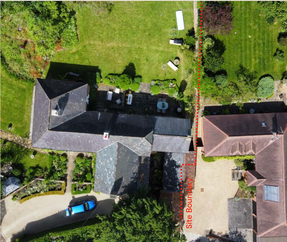
Figure 3- Aerial view of site and neighbouring property. The store roof is comprised of both slate and pantiles, divided over the site boundary.
