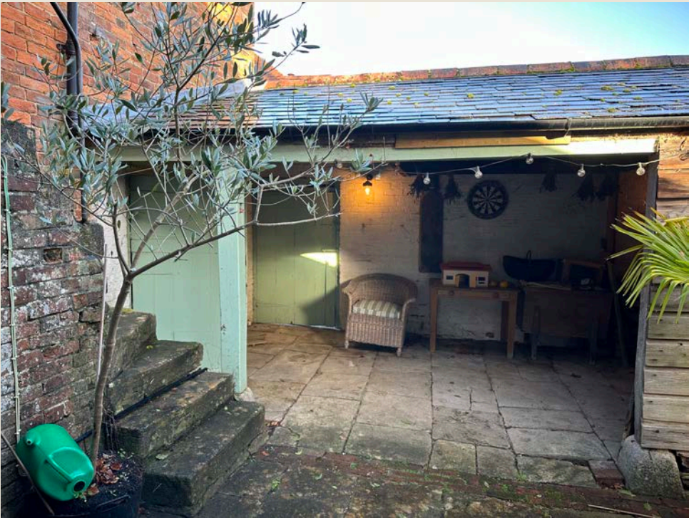
Figure 4 – View into store from courtyard
