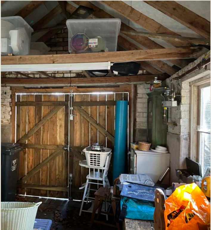
Figure 10- Garage doors along the east elevation of the garage. Roof has been replaced more recently
