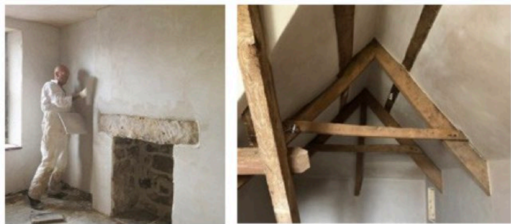
Hand trowelled Lime & Cork internal plaster finish
