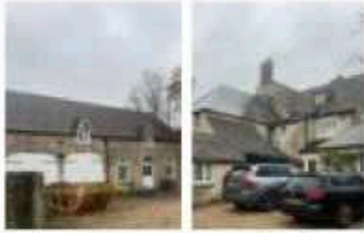
Oaksey House (Listed Building)
