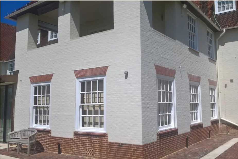
Example of proposed finish with lime shelter coat
