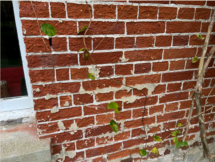
Figure 3– Exposed brickwork after paint removal
