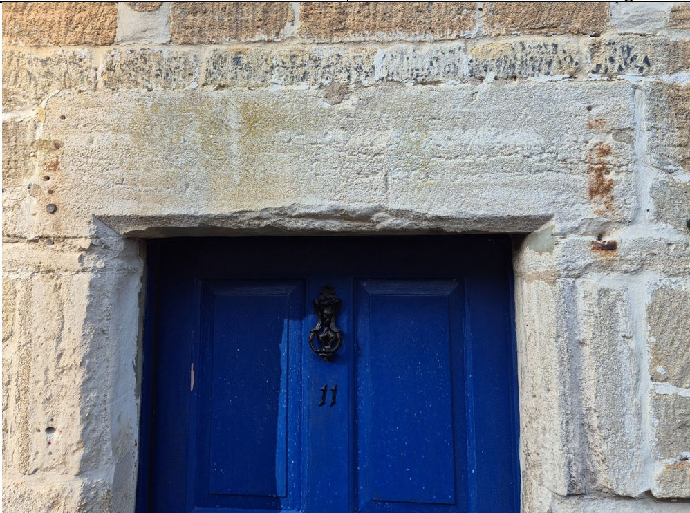
Evidence of iron fixings for earlier canopy
