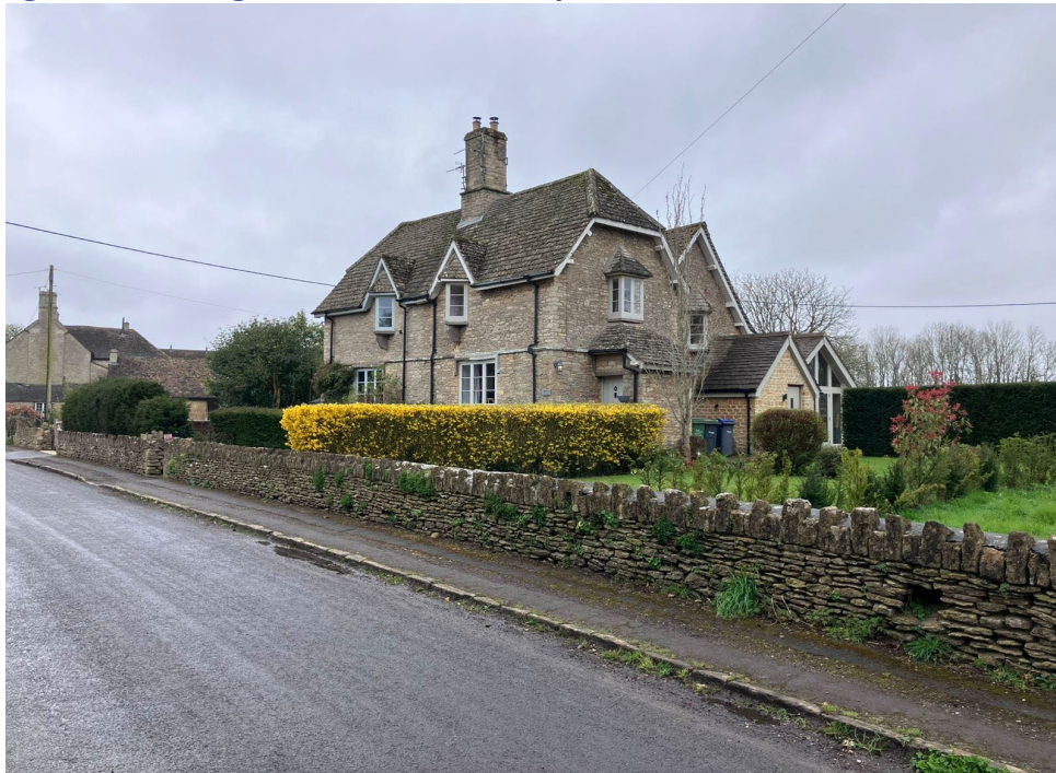
Fig.4 Rose Cottage – Garden/ boundary wall
