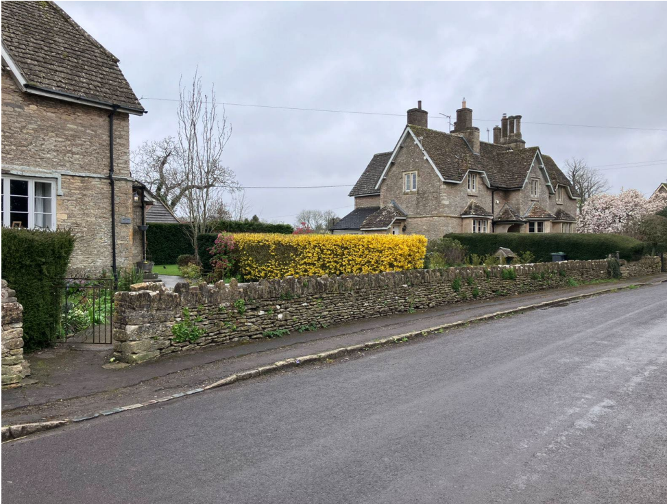
Fig.5 Rose Cottage – Garden/ boundary wall
