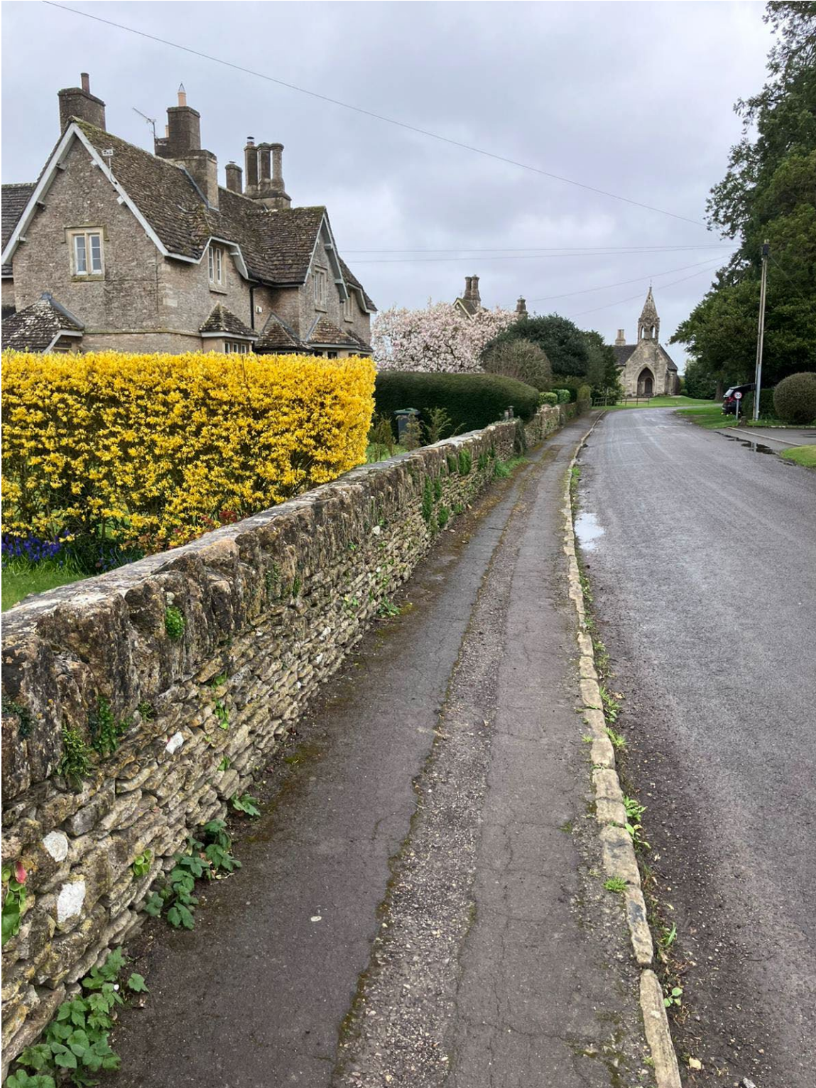
Fig.7 Rose Cottage – Good Visibility (North East direction)
