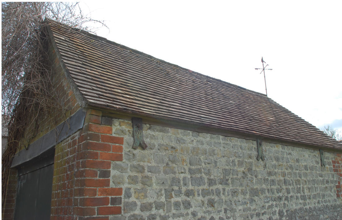
Figure 1 Plain clay tiled roof on adjacent outbuilding
