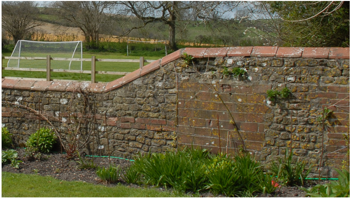
Figure 5 Brick and rubble garden wall to be reused i
