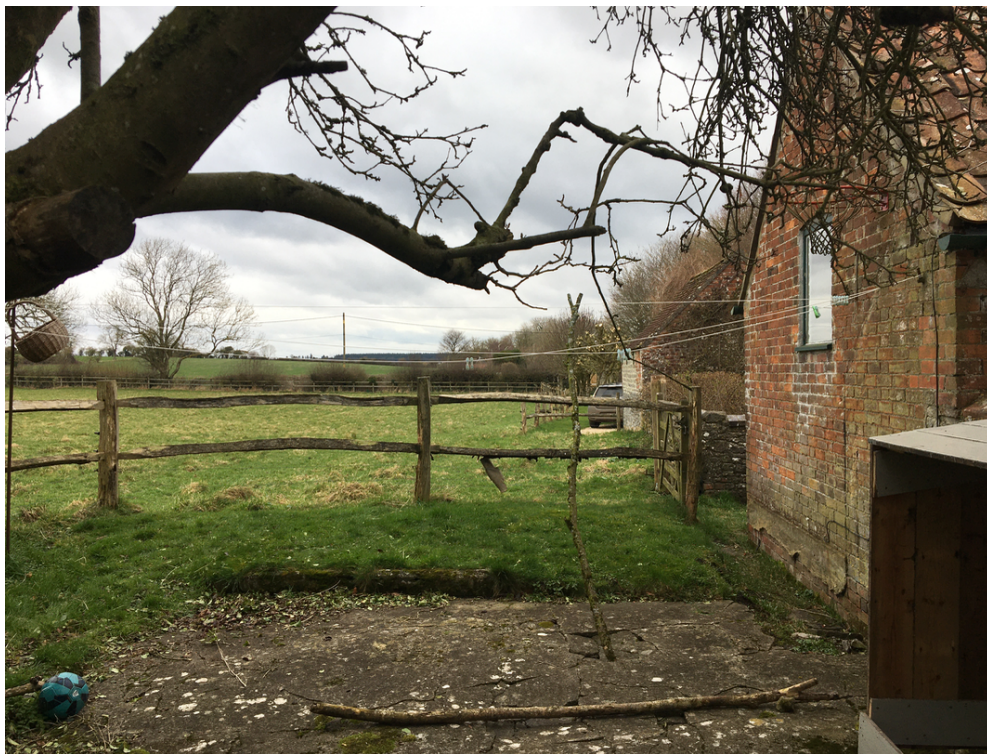
Figure 7 Concrete hard standing to be replaced with natural stone
