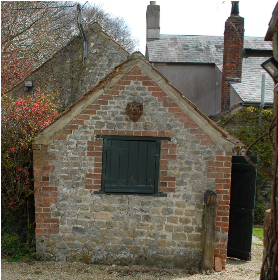
Figure 3 Decorative brick and rubble gable
