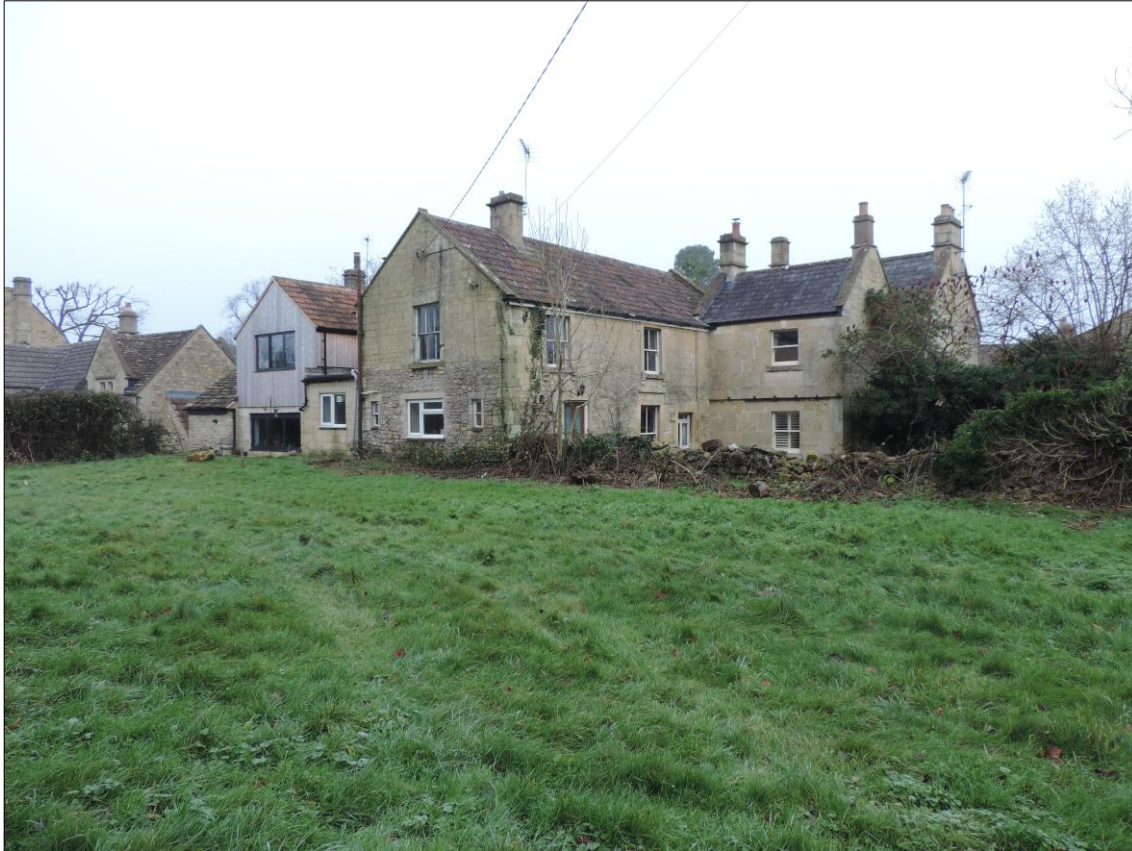
Photo 2 Northeast facing view from proposed development area towards no. 33 Winsley, with shared drystone wall in poor state of repair.
