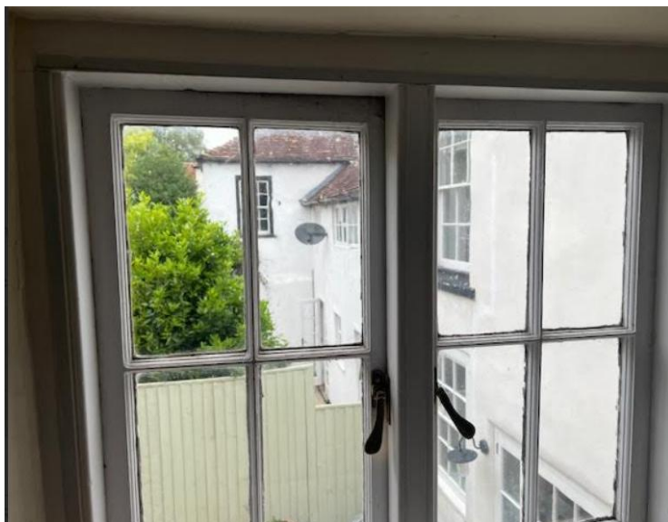
First floor window
