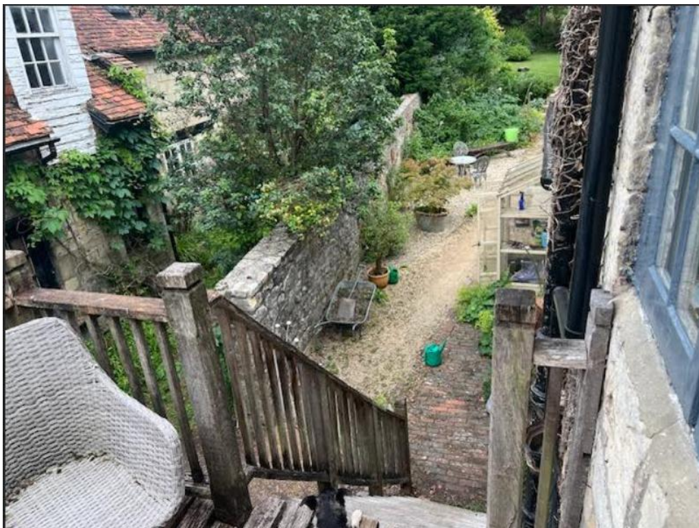
Existing stairs to be removed
