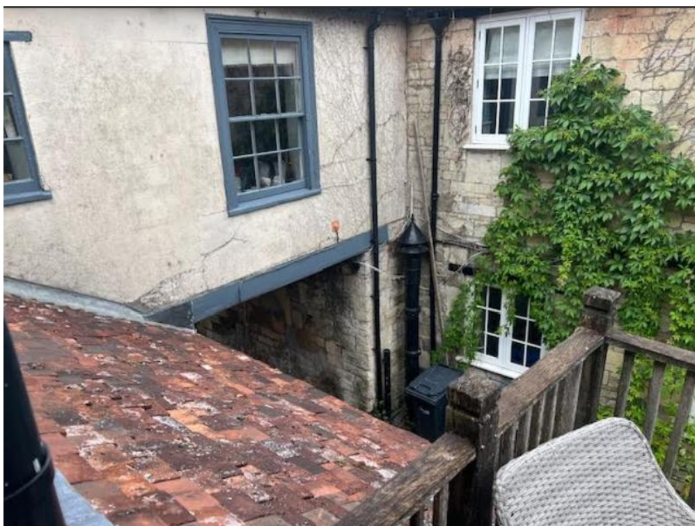
View from balcony towards shared access (to be removed)
