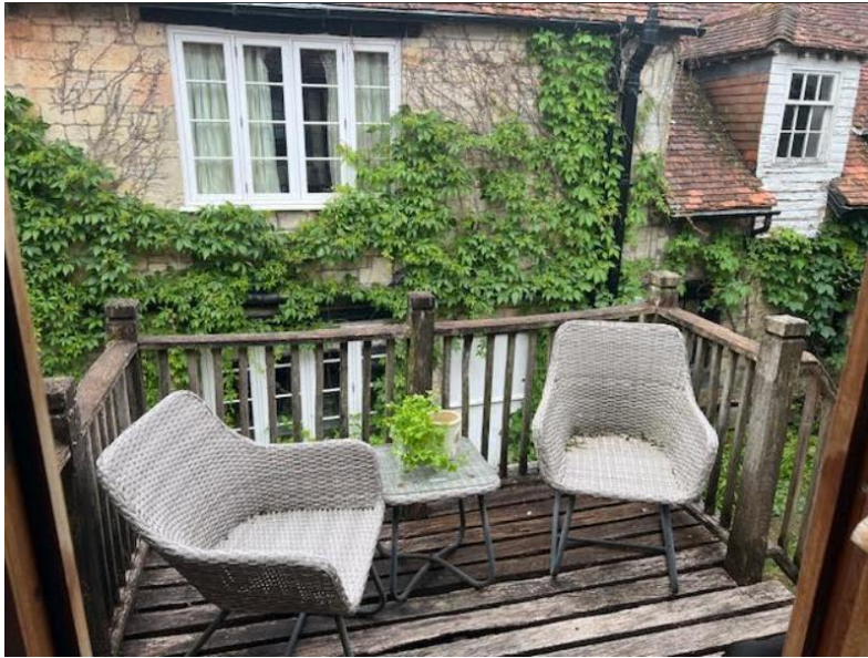
Balcony and stairs to be removed
