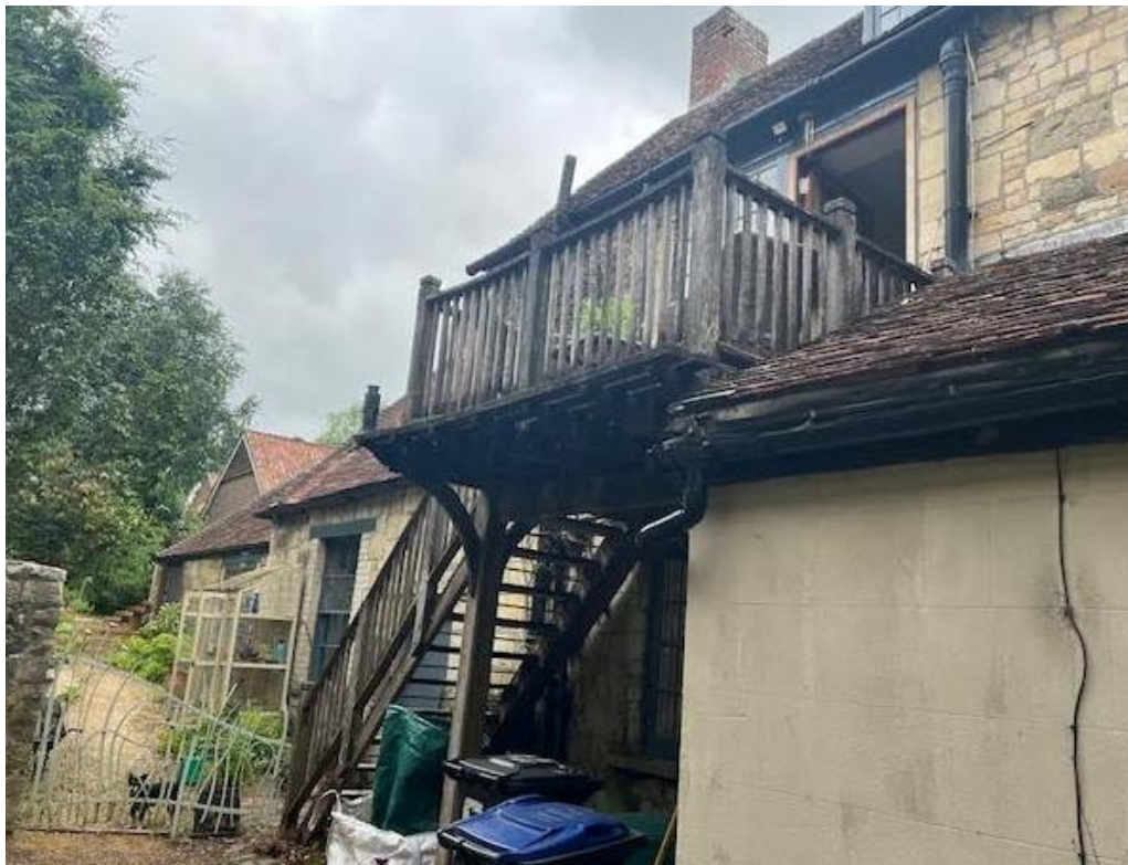
Figure 3 - External staircase to be removed
