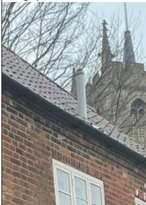
Fig. 4 Example of Soil Stack Already Installed On Westerly Elevation (at No.3 St Mary's Cottages)
