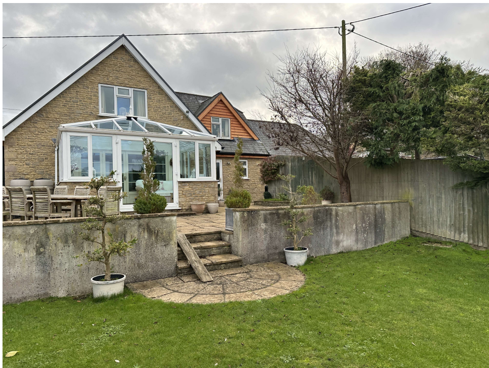
Photograph 04, Existing rear elevation of existing dwelling showing conservatory.
