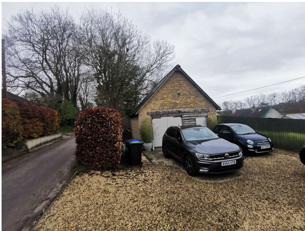
Photograph 02, Existing outbuilding front elevation from driveway.
