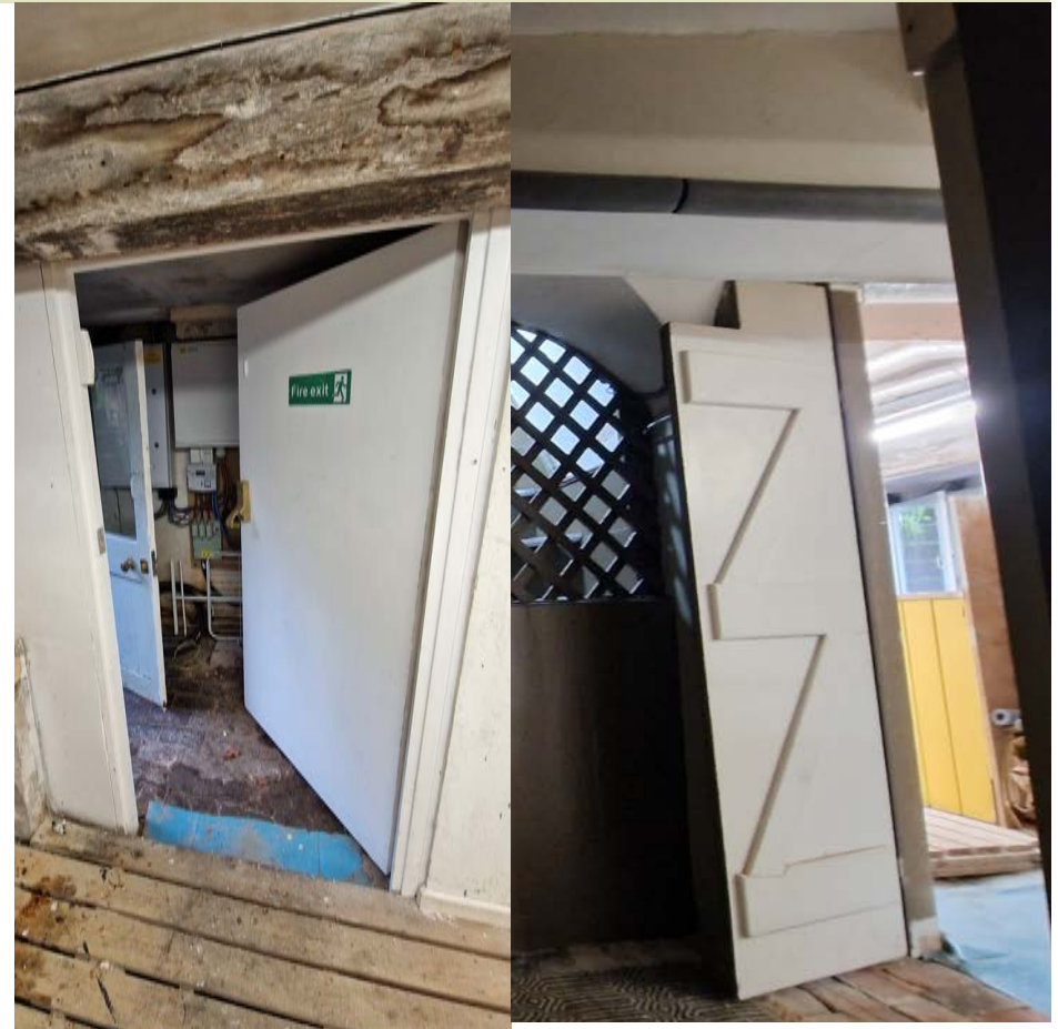
Modern doors and partitions on the east side of the basement to be removed
