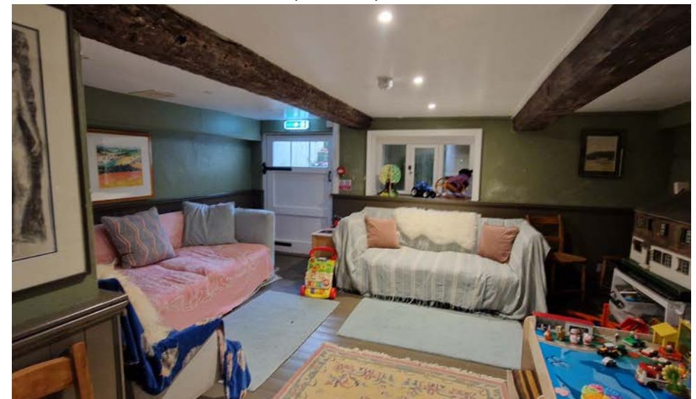
West side of basement recently repaired -retaining joinery
