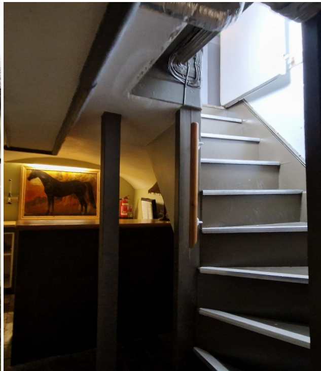
Shrewton House: internal alterations to Basement
