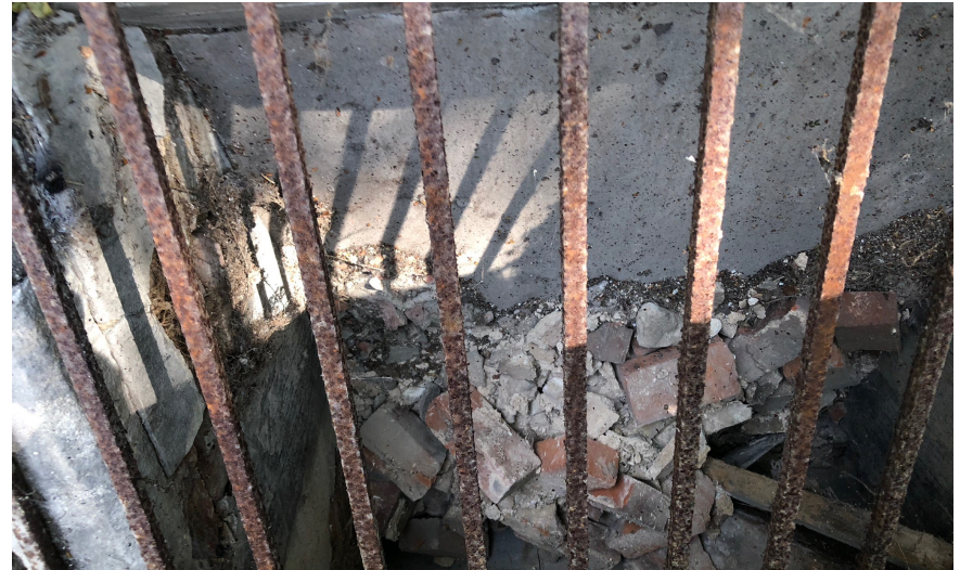
Blocked Light shafts since opened up.
