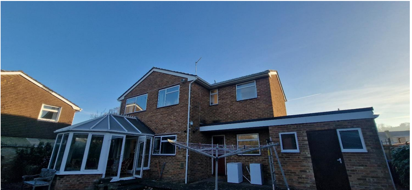
Picture 2: Showing the rear elevation
