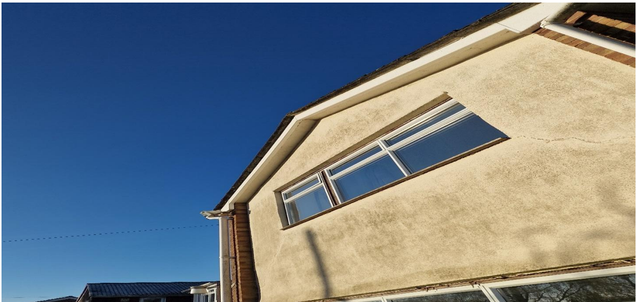
Picture 5: Showing tight fitting eaves
