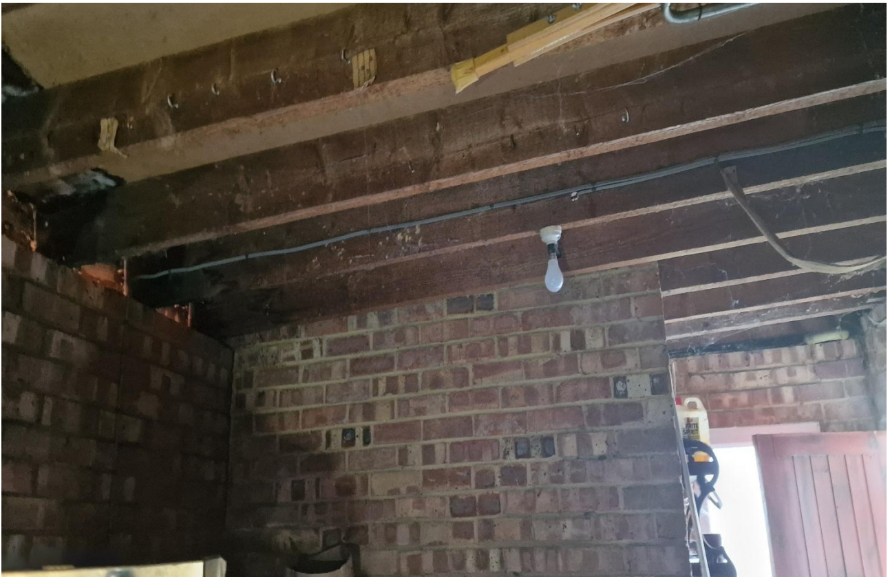
Picture 9: Showing the internal structure of the garage
