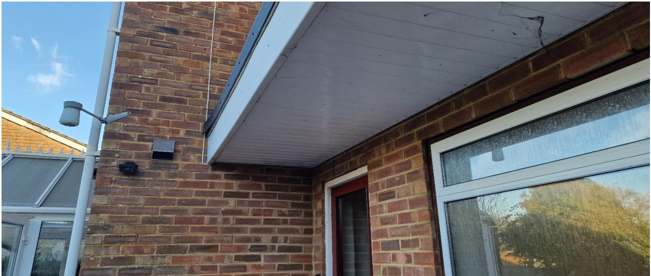
Picture 4: Showing the tight eaves
